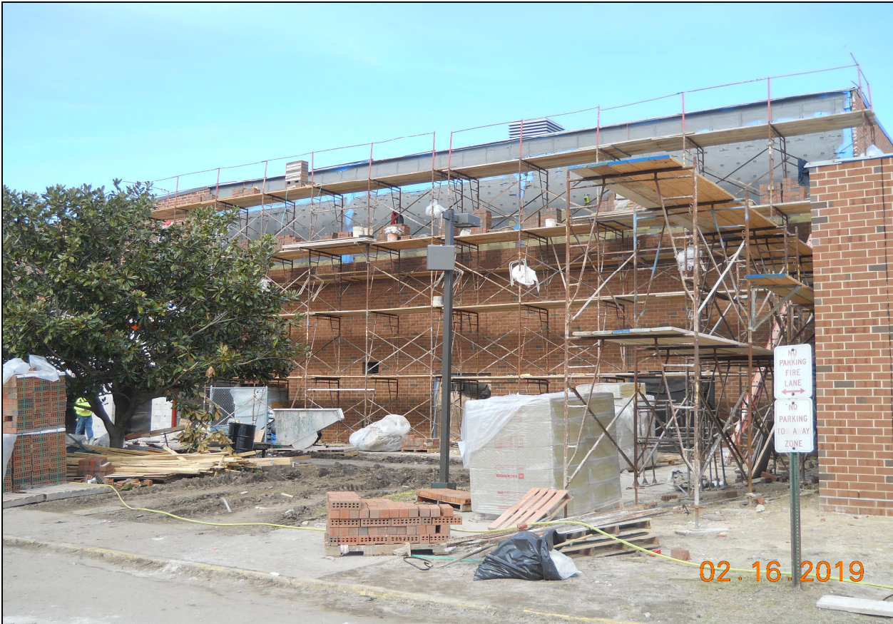
Pinelands Regional Sr. High School 6 Exterior Masonry Installation (West D-Block & Auditorium)
