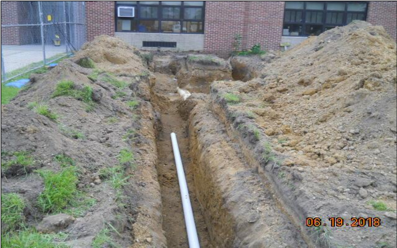
Pinelands Modular Classrooms – Underground Plumbing
