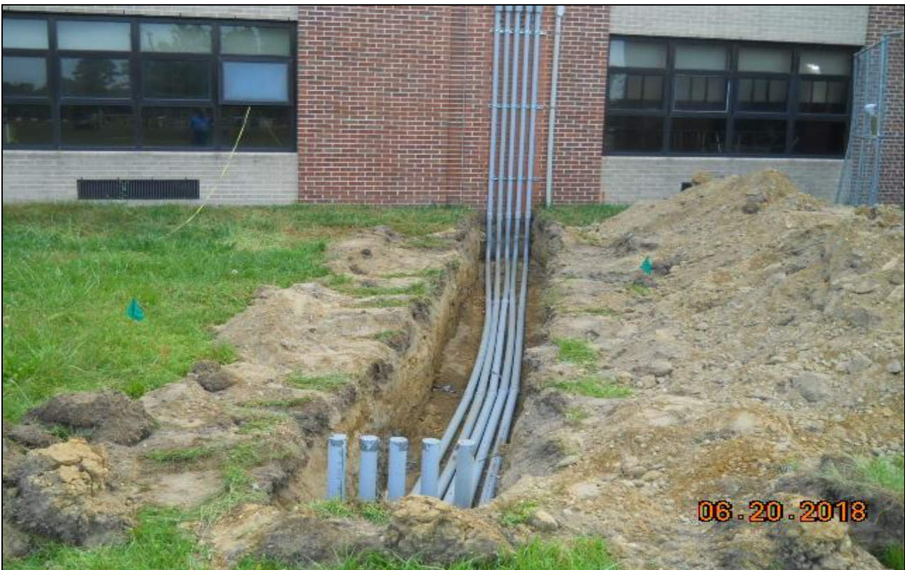
Pinelands Regional Modular Classrooms – Underground Electrical Conduit
