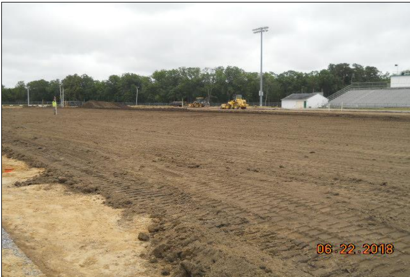
Pinelands Regional Athletic Field – Topsoil Preparation
