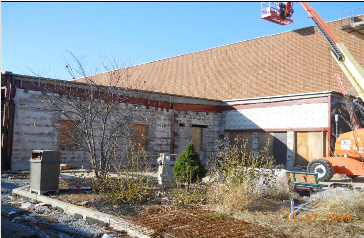
Pinelands Regional Sr. High School 6 Exterior Masonry Waterproofing / Brick Veneer Installation
