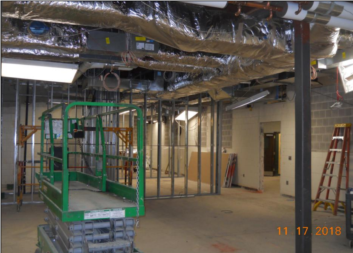
Pinelands Regional Sr. High School 6 Main Office Renovation (Wall Framing)
