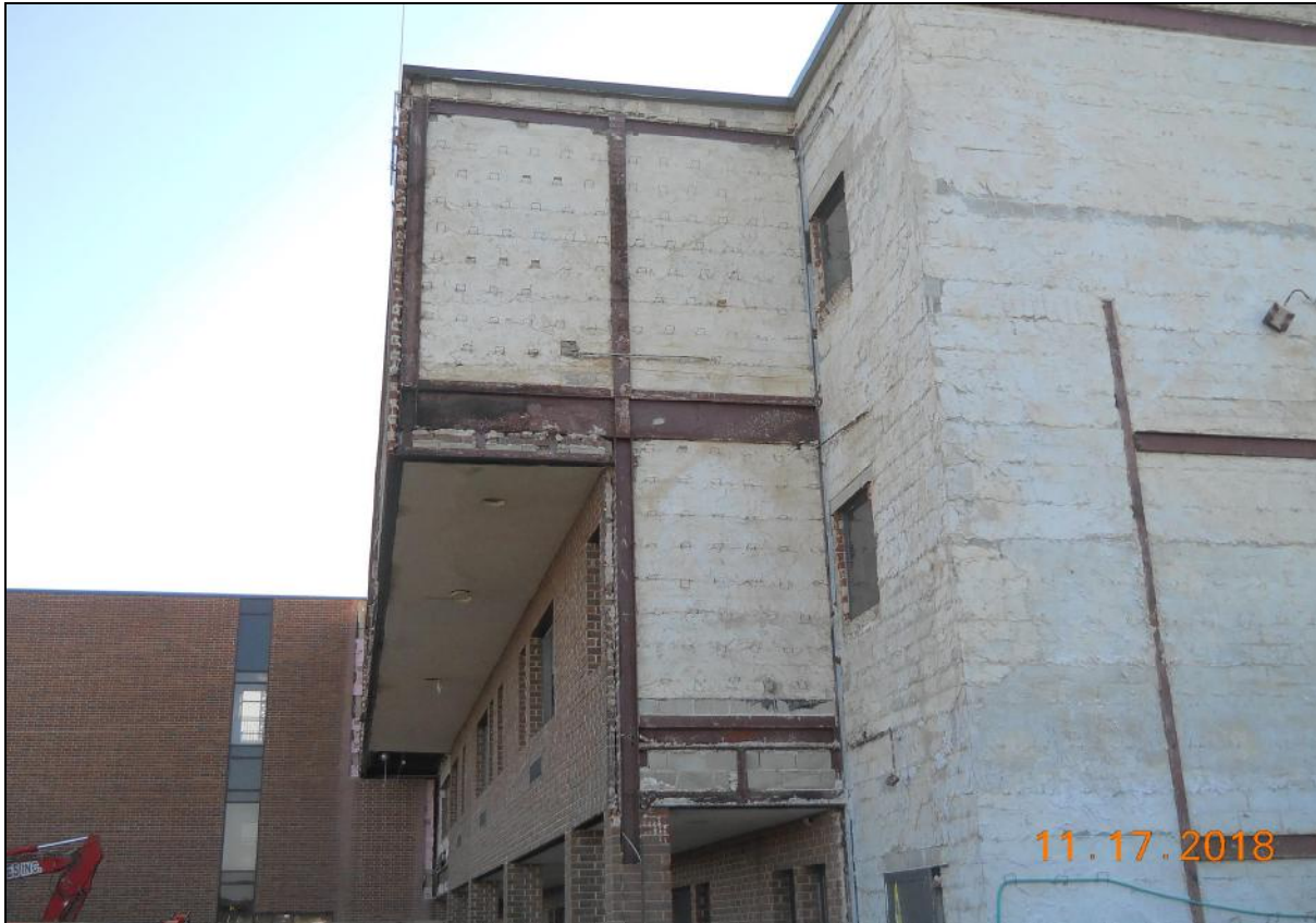
Pinelands Regional Sr. High School 6 Exterior Masonry Facia Demolition (A-Wing)
