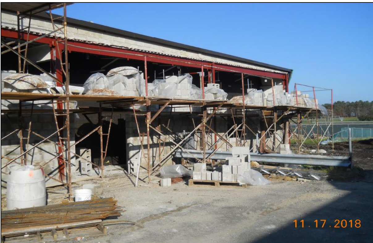
Pinelands Regional Sr. High School 6 Exterior Masonry Wall Installation D-Wing East
