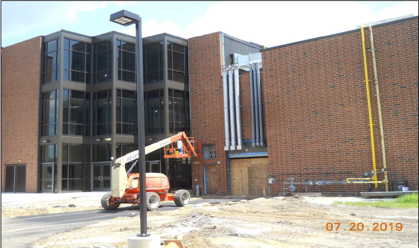
Pinelands Regional Sr. High School 6 Heating Plant Vent Piping Installation (Block A South 6 Boiler Room)
