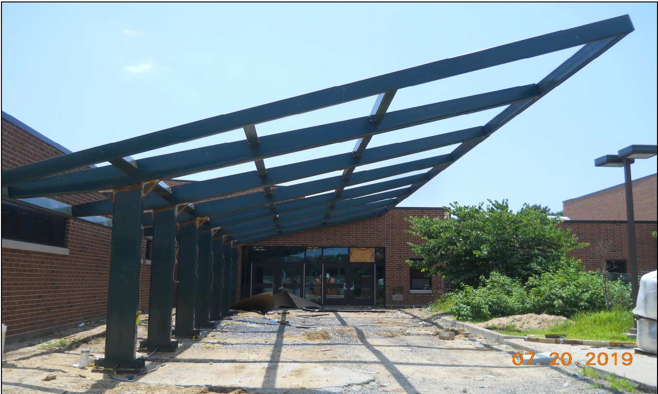
Pinelands Regional Sr. High School 6 Completed Entrance Canopy Steel Structure Installation
