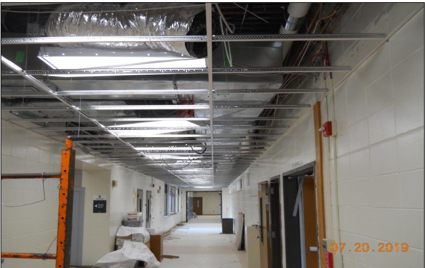
Pinelands Regional Jr. High School 6 Ceiling System Grid Installation (B Corridor)
