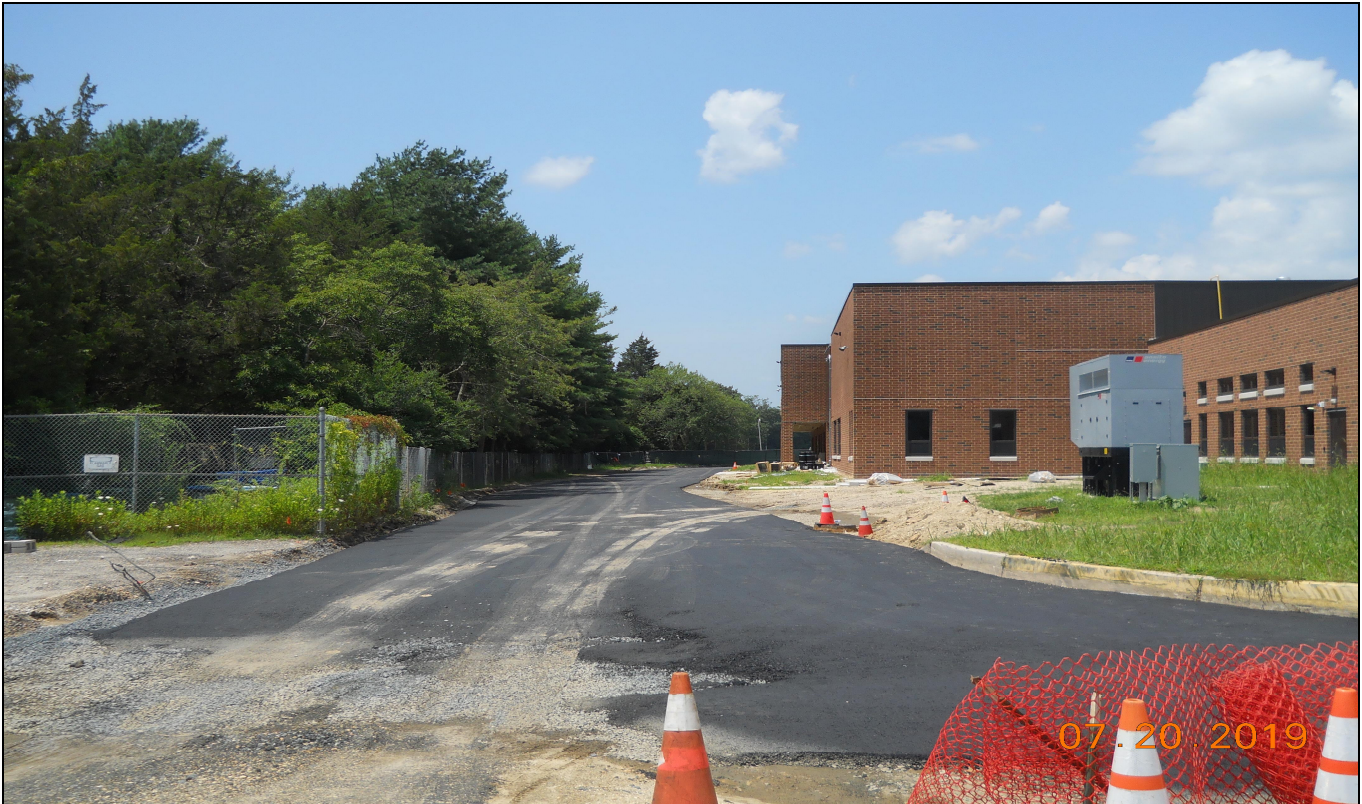
Pinelands Regional Sr. High School 6 Rear Service Road Base-Pavement Installation
