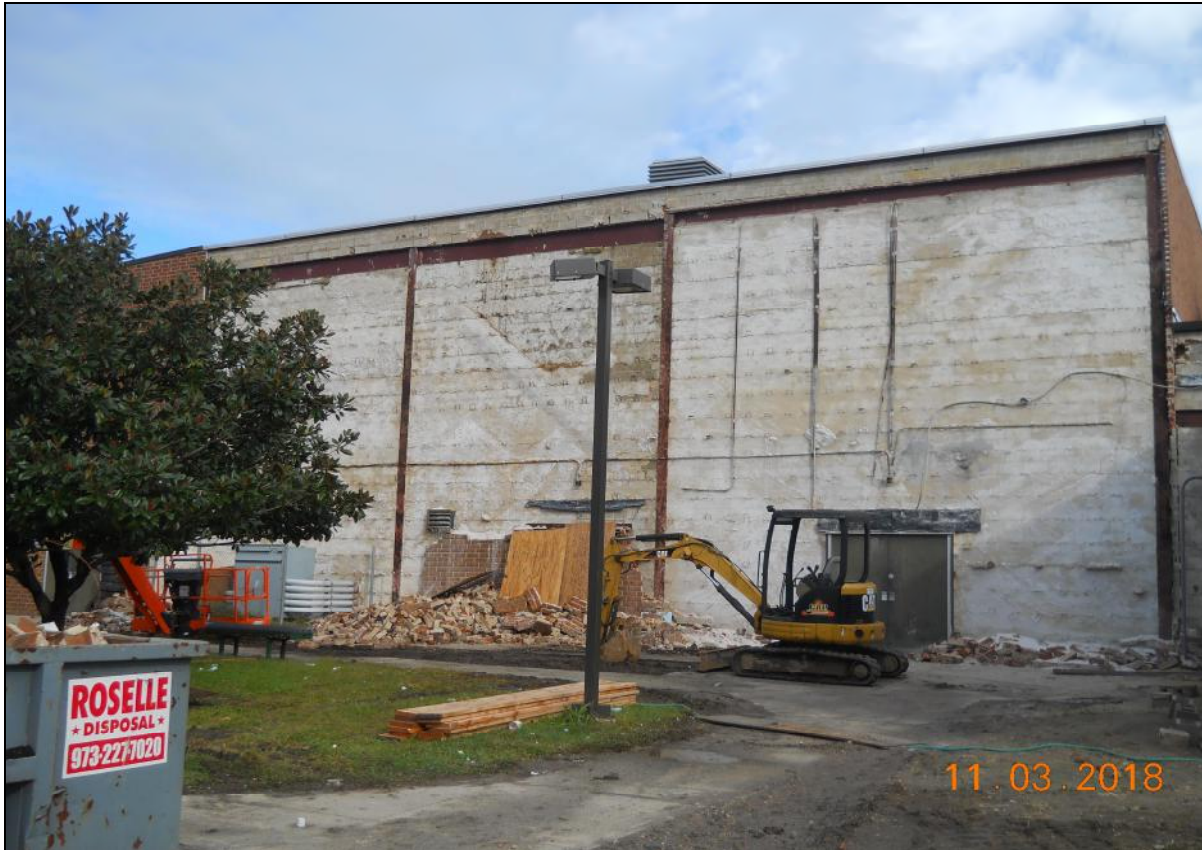
Pinelands Regional Sr. High School 6 Exterior Masonry Facia Demolition Auditorium
