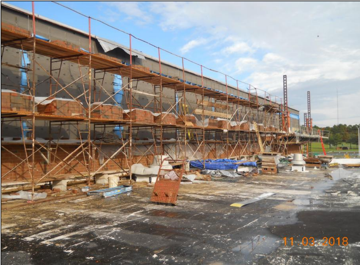
Pinelands Regional Sr. High School 6 Exterior Masonry Waterproofing / Brick Veneer Installation
