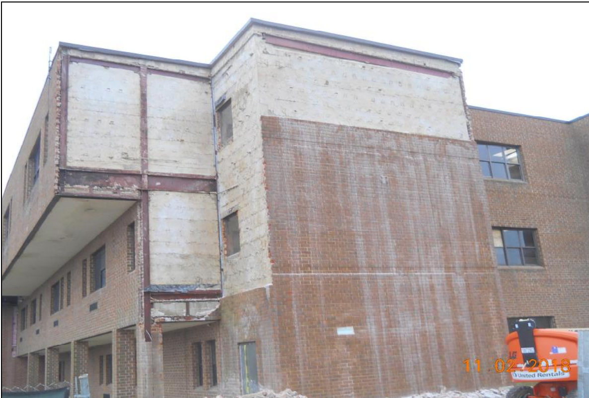
Pinelands Regional Sr. High School 6 Exterior Masonry Facia Demolition A-Wing West
