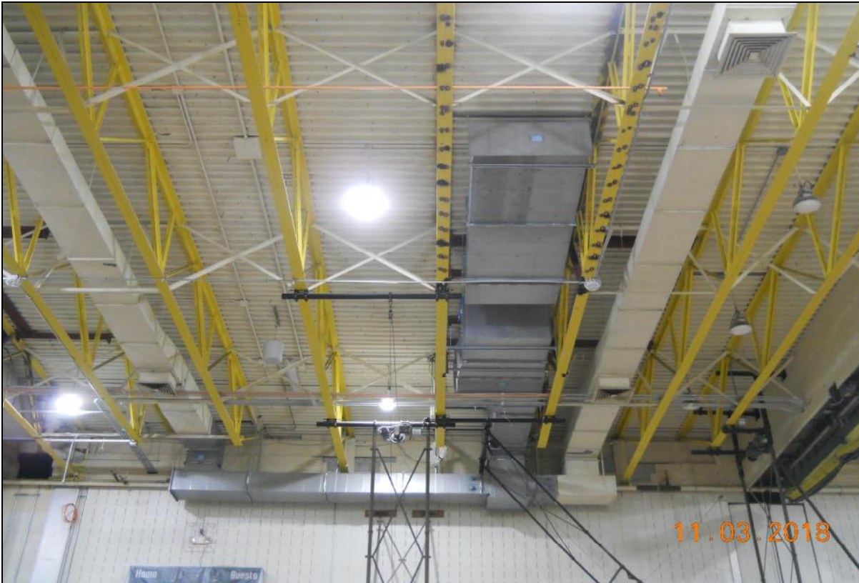
Pinelands Regional Sr. High School 6 New HVAC Ductwork GYM
