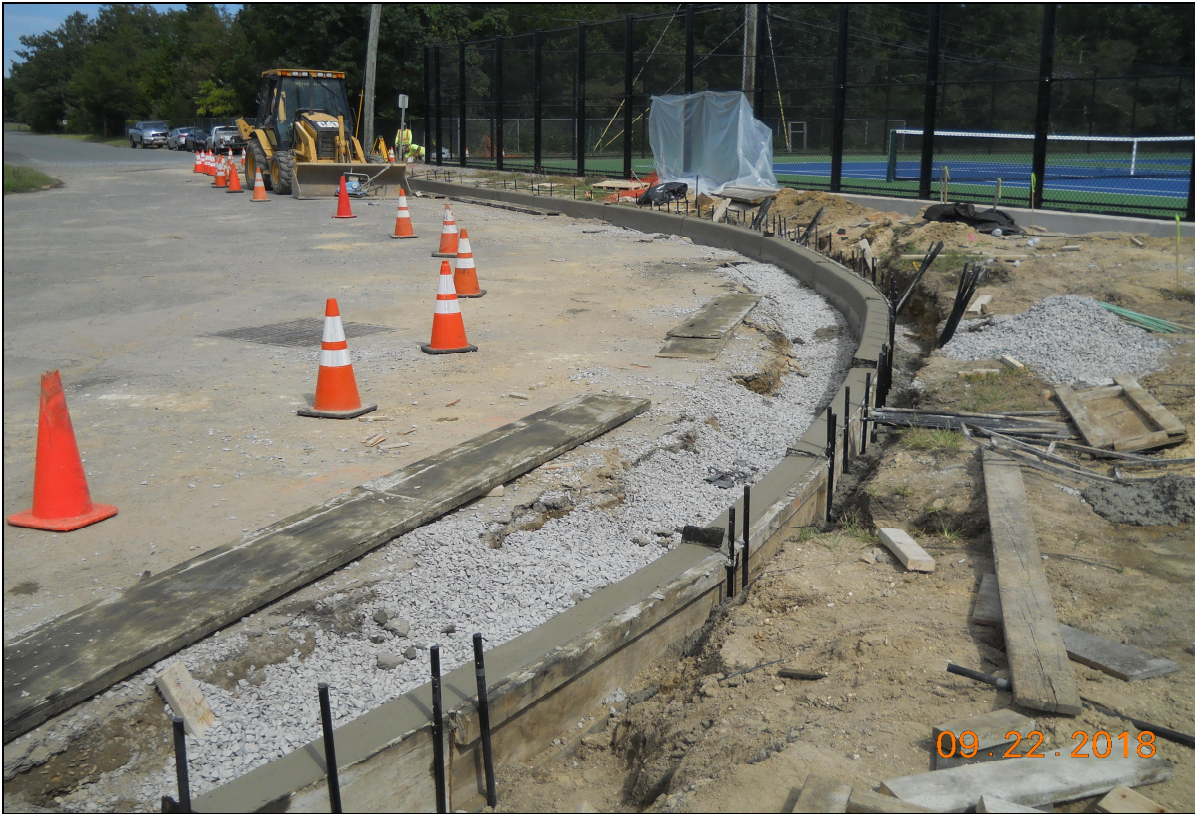
Pinelands Regional Tennis Courts ó Sidewalk & Curbing Installation
