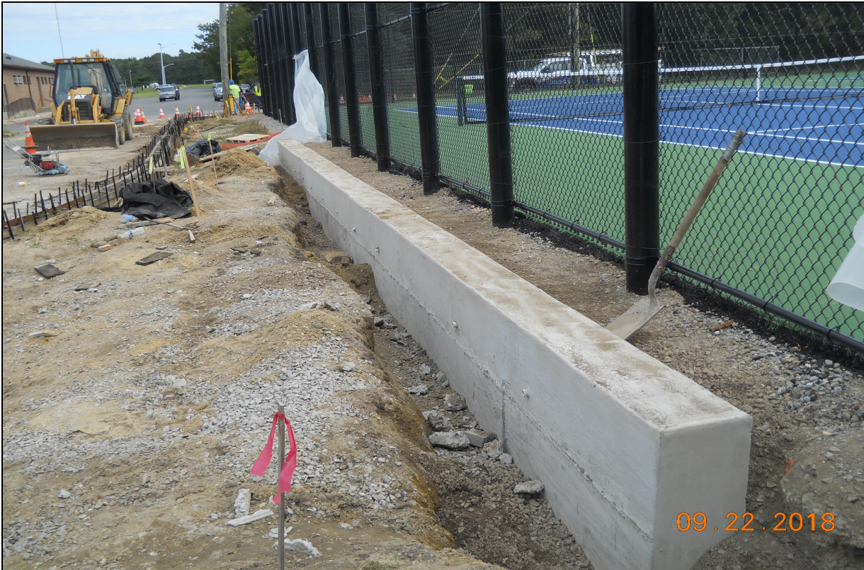
Pinelands Regional Tennis Courts 6 Retaining wall Installation
