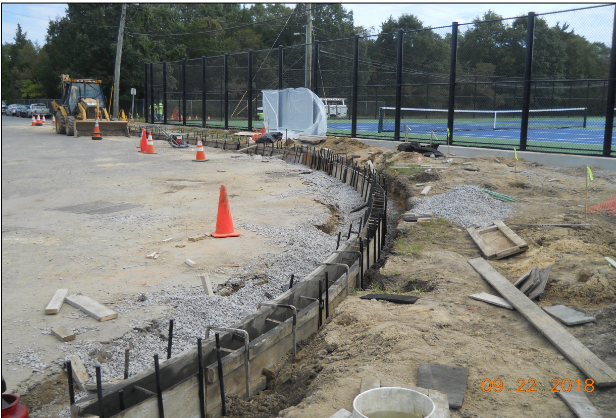
Pinelands Regional Tennis Courts 6 Sidewalk & Curbing Installation
