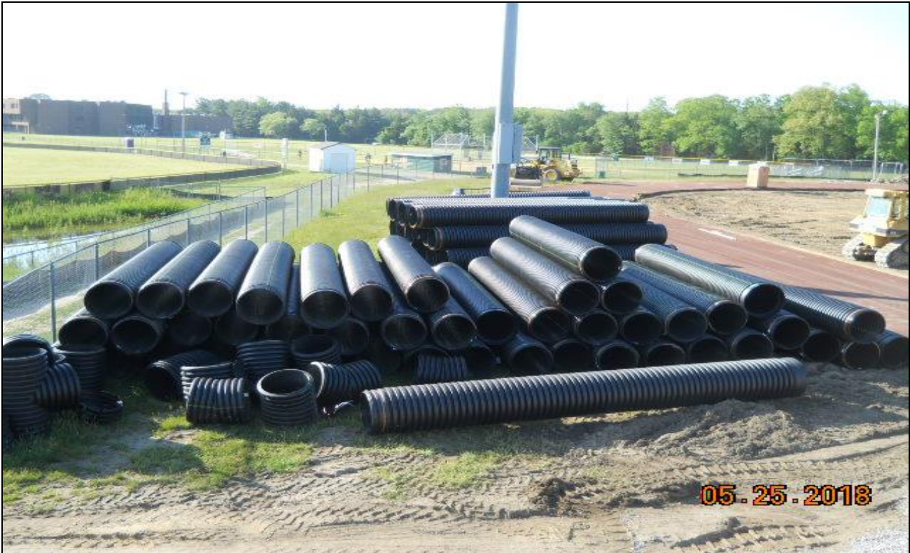
Pinelands Regional Athletic Field – Drainage System Piping
