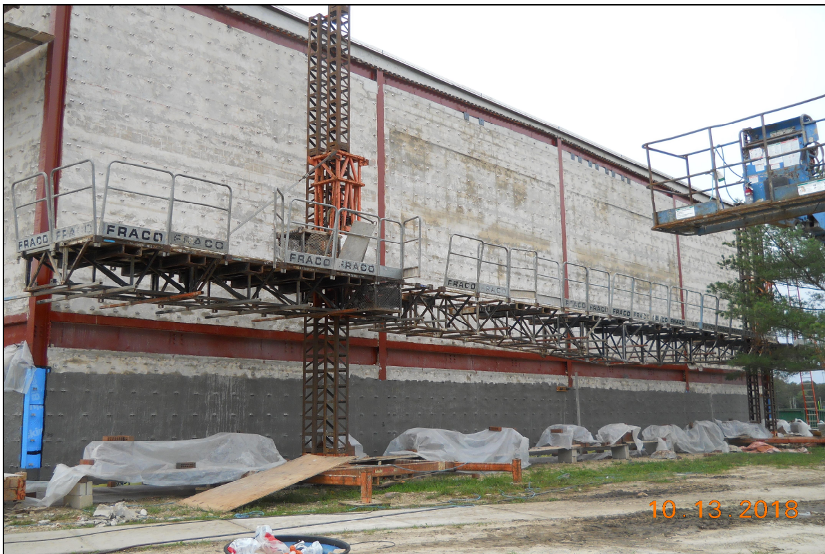
Pinelands Regional Sr. High School 6 Exterior Masonry Waterproofing / Brick Veneer Installation
