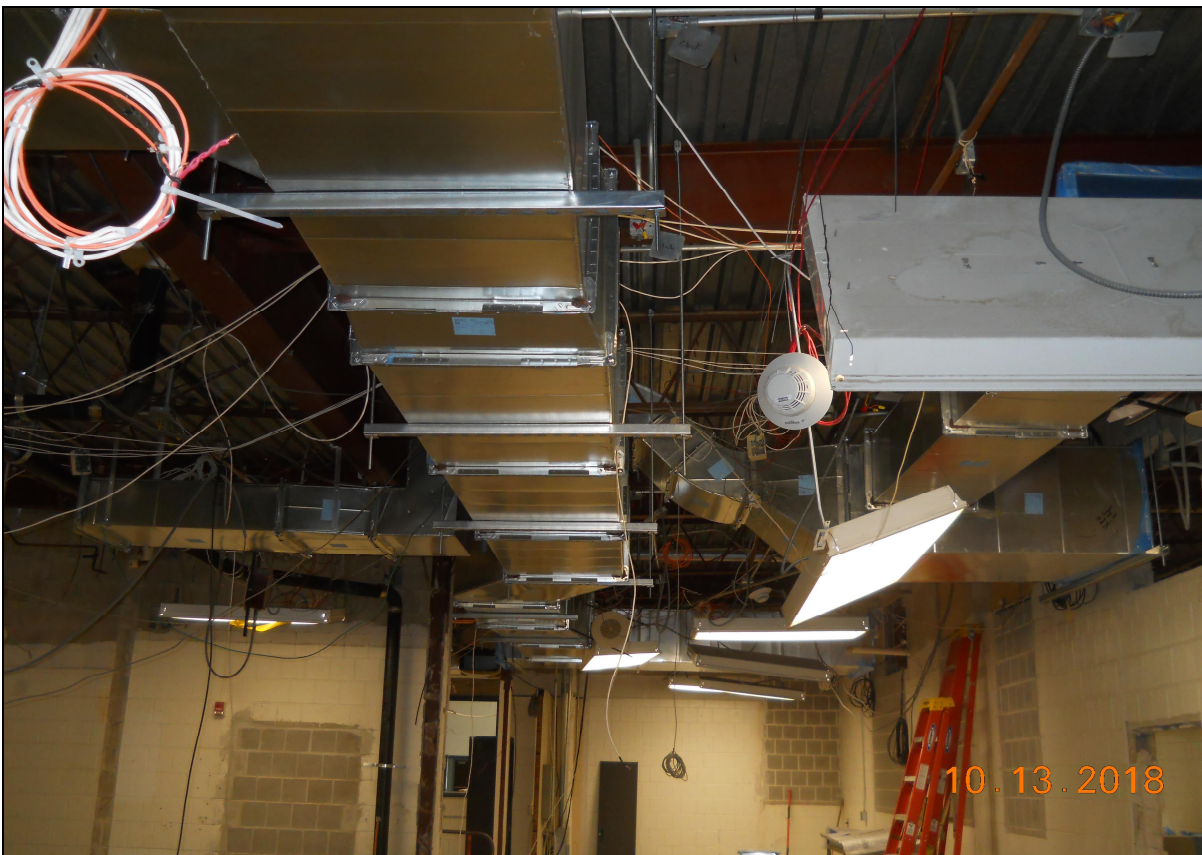
Pinelands Regional Sr. High School 6 Main Office HVAC Ductwork Installation
