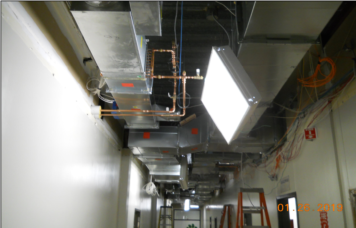
Pinelands Regional Sr. High School 6 (A-Block) HVAC Ductwork
