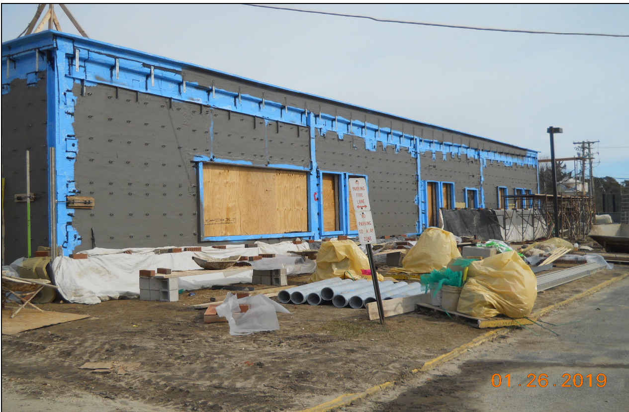
Pinelands Regional Sr. High School 6 Exterior Masonry & Waterproofing (D-Wing South)
