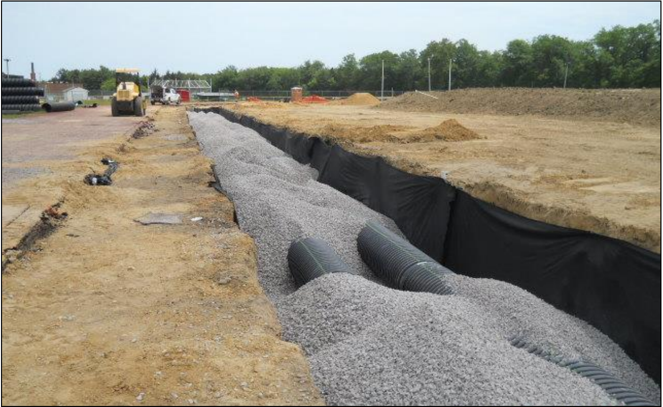
Pinelands Regional Athletic Field – Drainage System Installation
