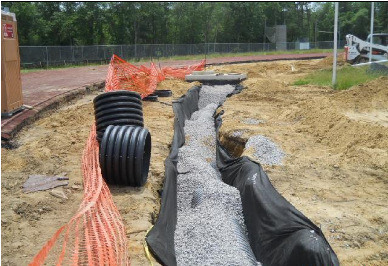
Pinelands Regional Athletic Field – Drainage System Installation
