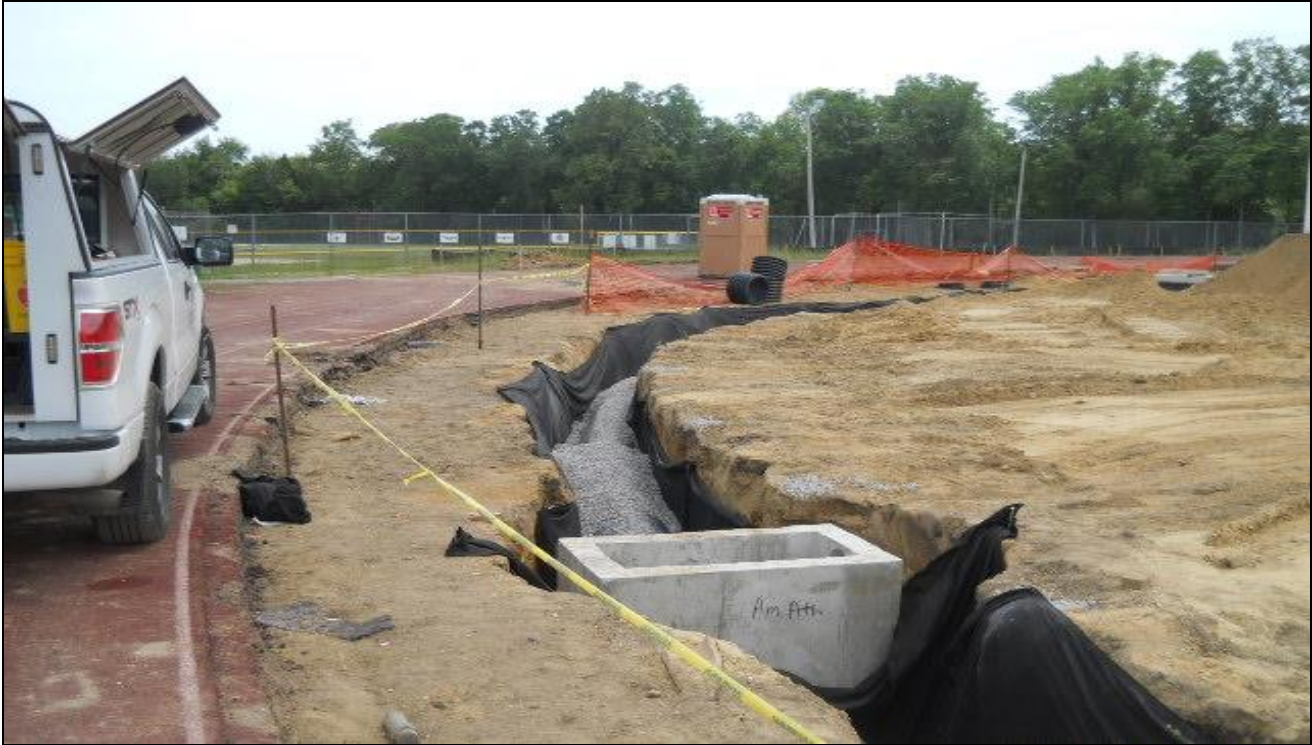
Pinelands Regional Athletic Field – Drainage System Installation
