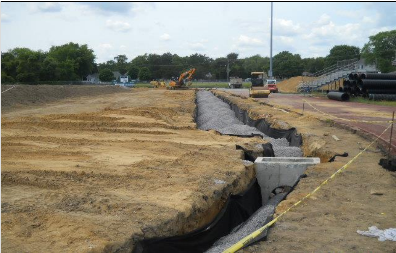
Pinelands Regional Athletic Field – Drainage System Installation
