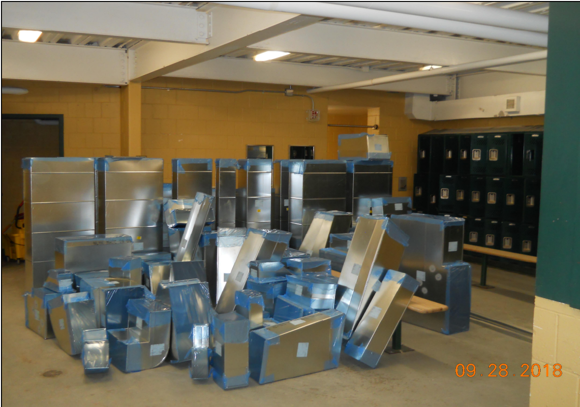
Pinelands Regional Sr. High School 6 Locker Room HVAC Ductwork (New)
