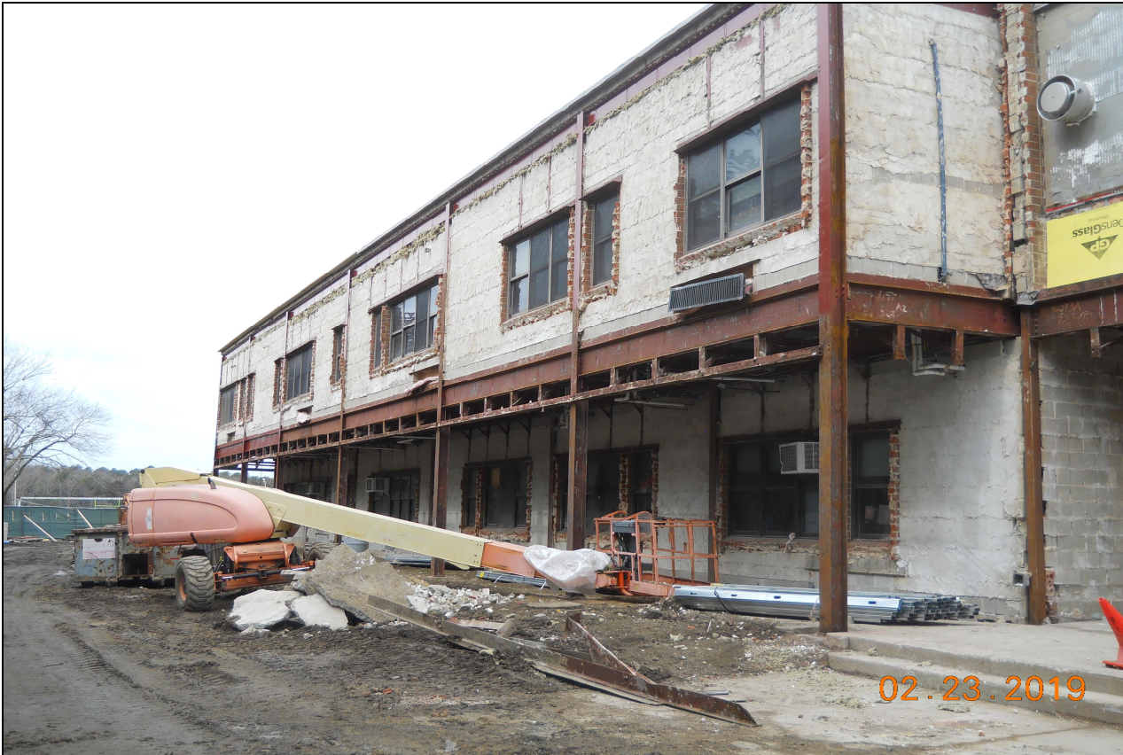
Pinelands Regional Sr. High School 6 Exterior Masonry Facia Demolition & Preparation (A Block - South)
