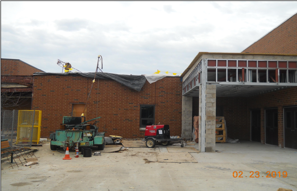
Pinelands Regional Sr. High School 6 Exterior Masonry Installation (Gym Entrance)
