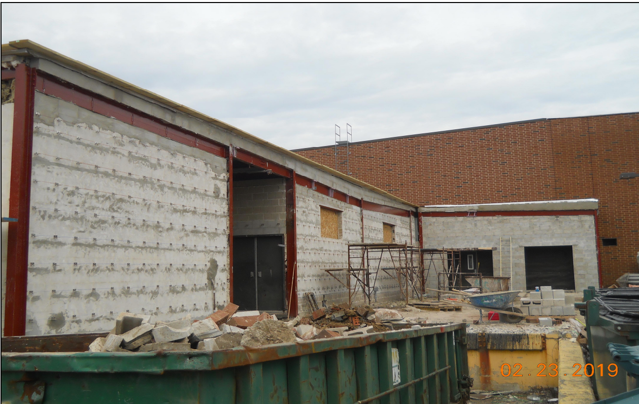
Pinelands Regional Sr. High School 6 Exterior Wall Reconstruction & Preparation (C Block East)
