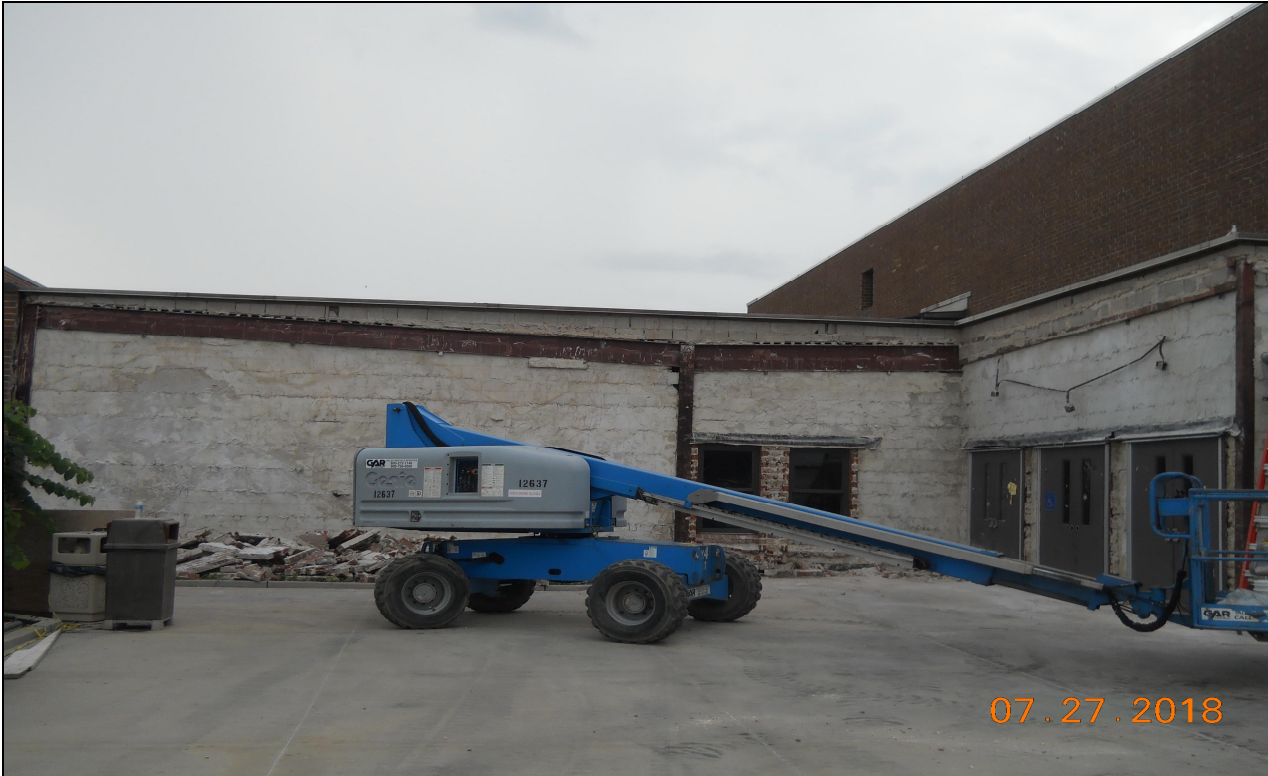
Pinelands Regional Sr. High School 6 Exterior Brick Fascia Removal
