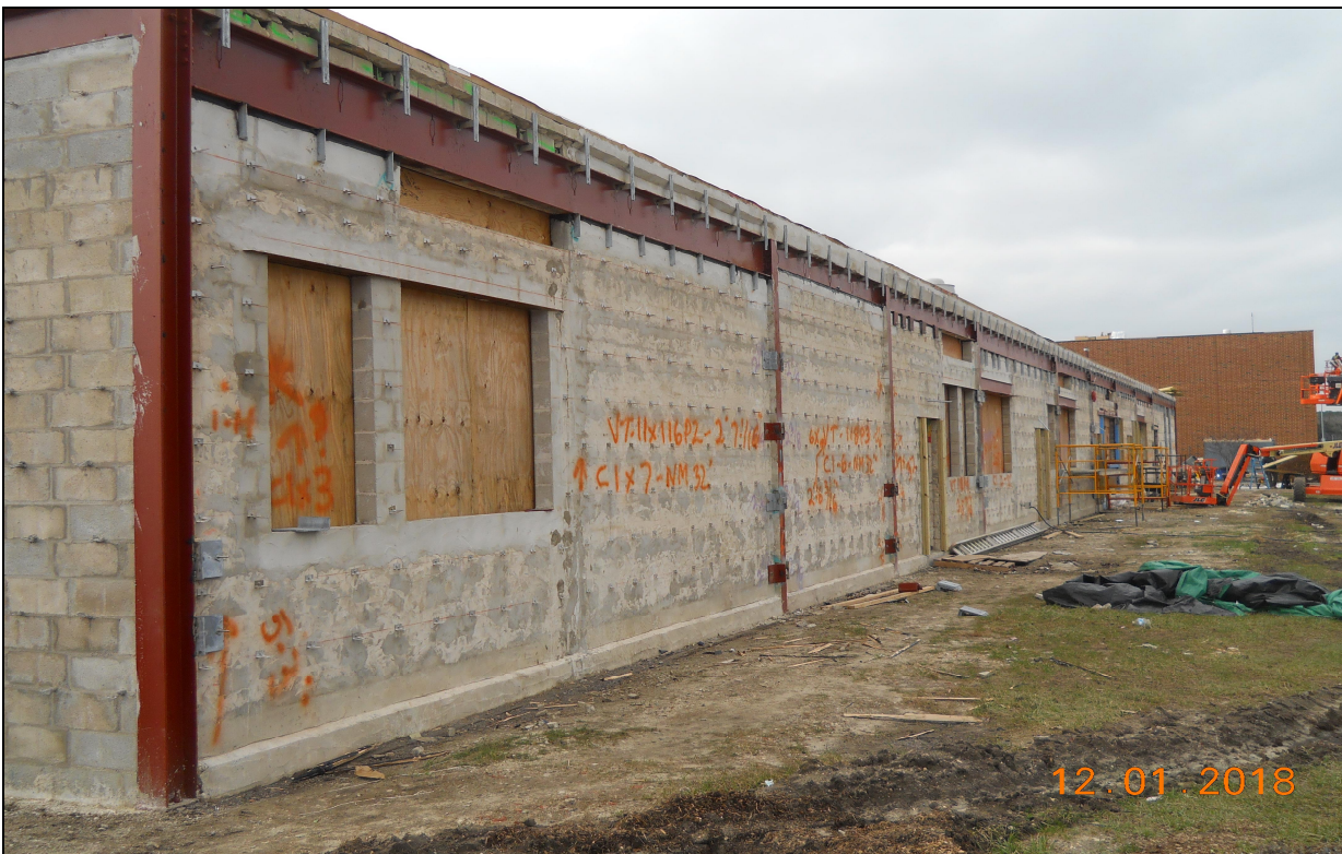
Pinelands Regional Sr. High School □ Exterior Masonry / Steel Installation (D-Wing East)
