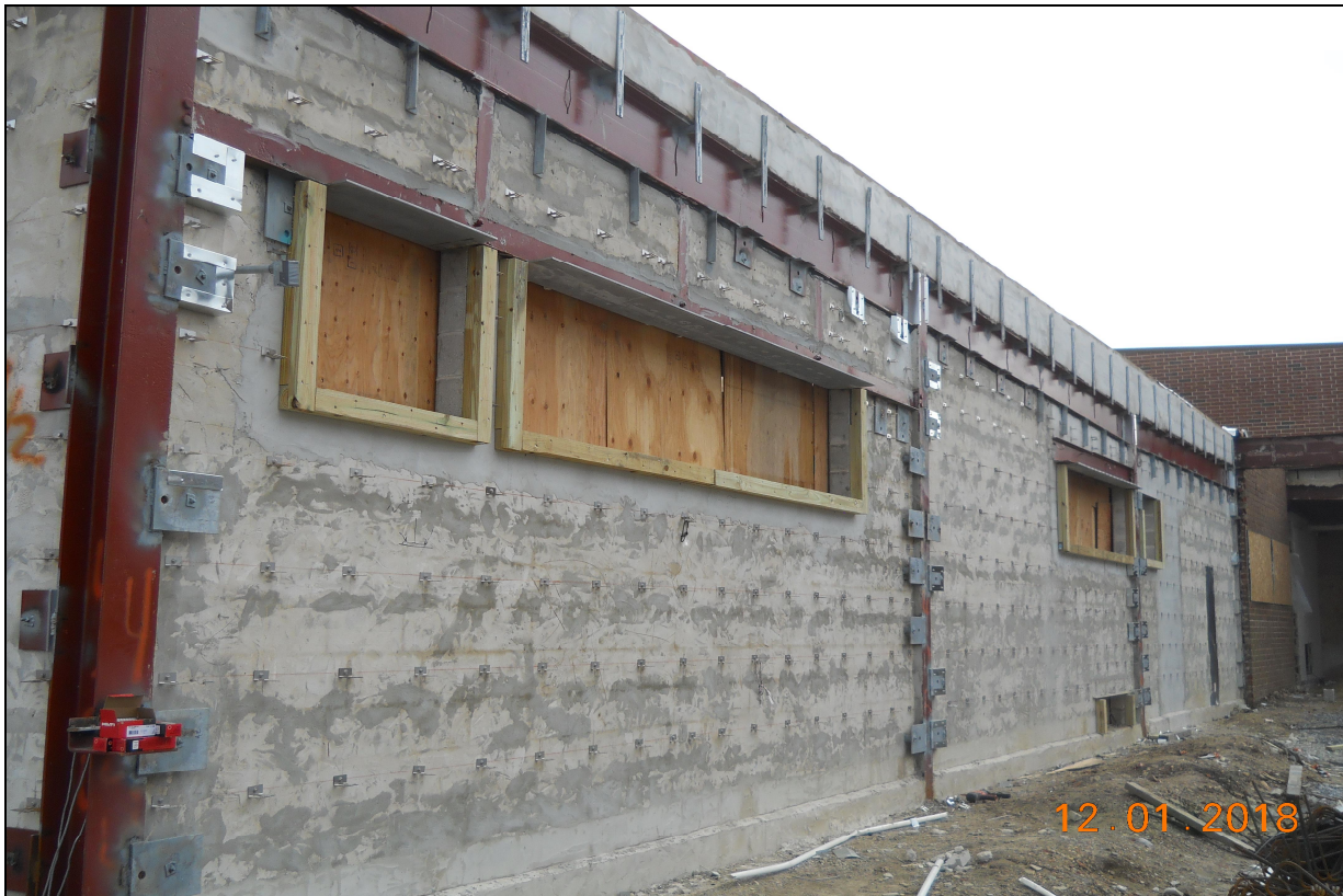
Pinelands Regional Sr. High School □ Exterior Masonry / Steel Installation (D-Wing East)
