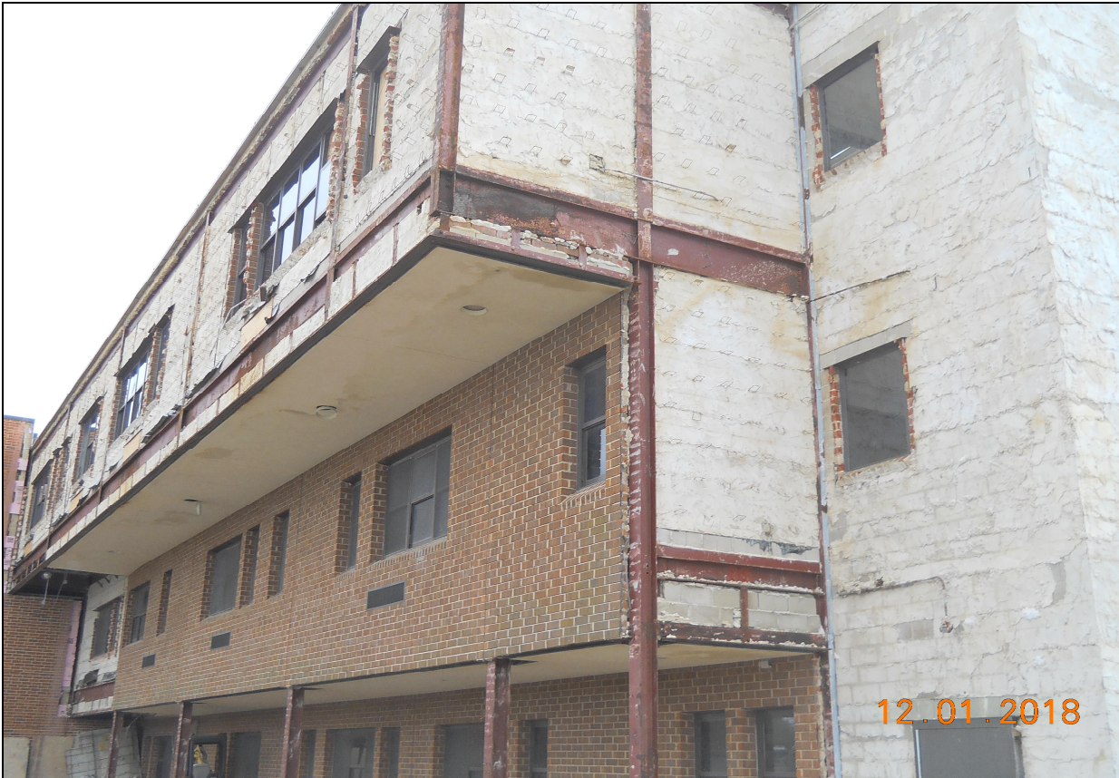
Pinelands Regional Sr. High School □ Exterior Masonry Facia Demolition (A-Wing)
