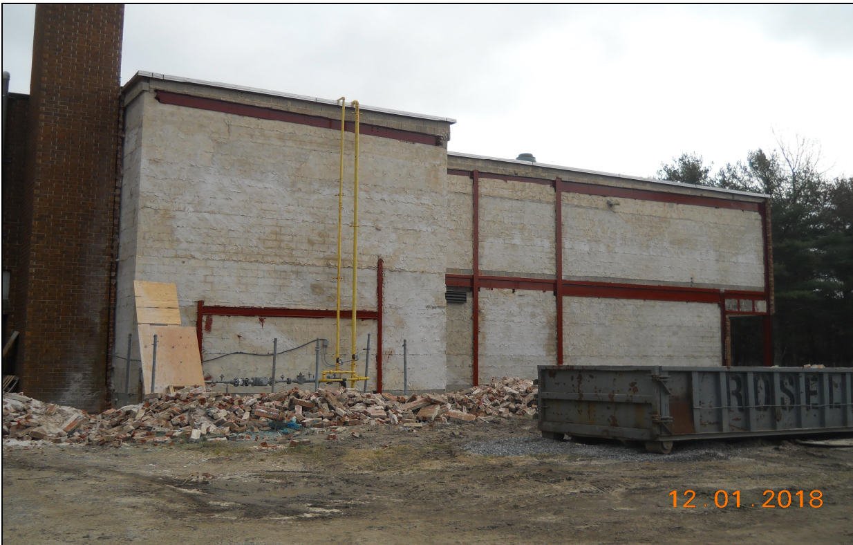
Pinelands Regional Sr. High School □ Exterior Masonry Facia Demolition (A-Wing)
