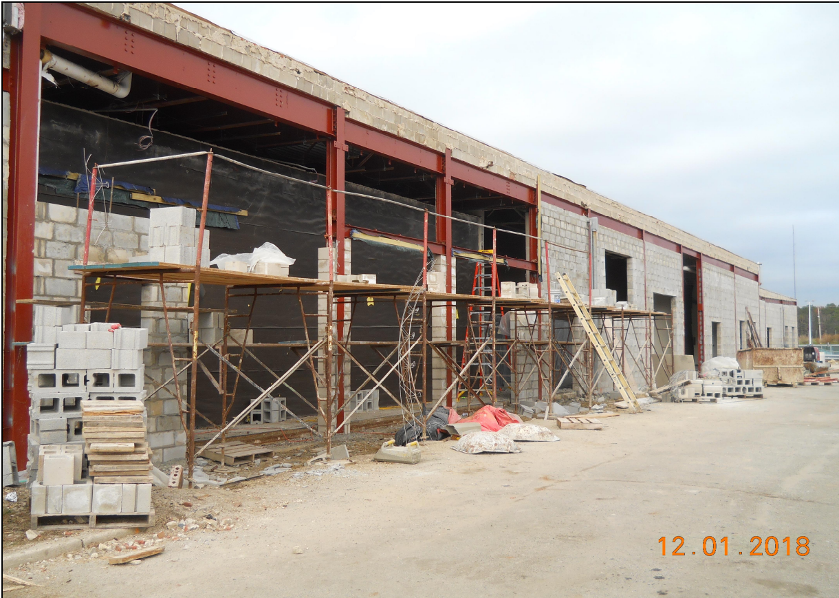
Pinelands Regional Sr. High School □ Exterior Masonry Installation (D-Wing East)
