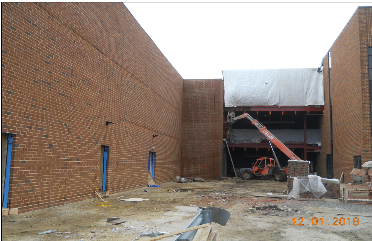
Pinelands Regional Sr. High School □ Exterior Masonry Waterproofing / Brick Veneer Installation
