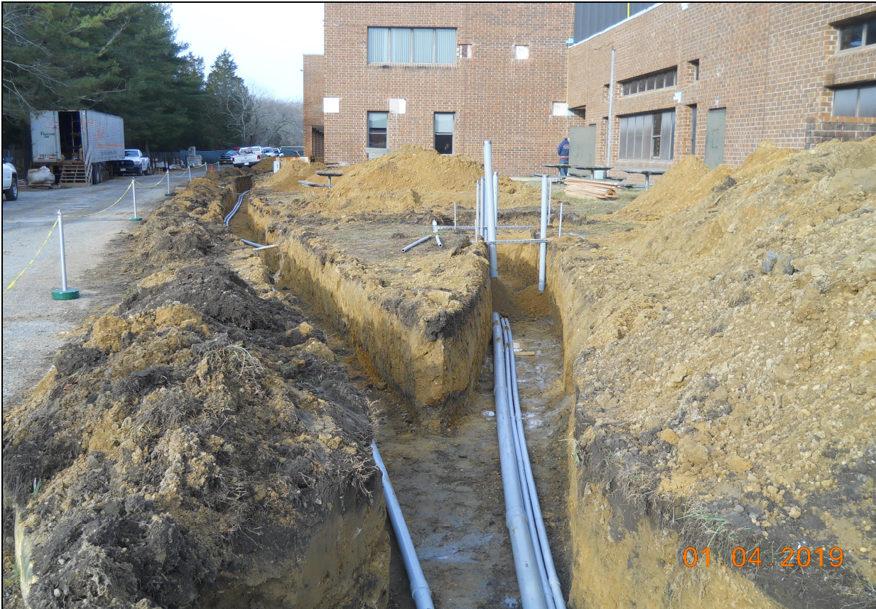
Pinelands Regional Sr. High School 6 Underground Elec. Conduit for New Emergency Generator
