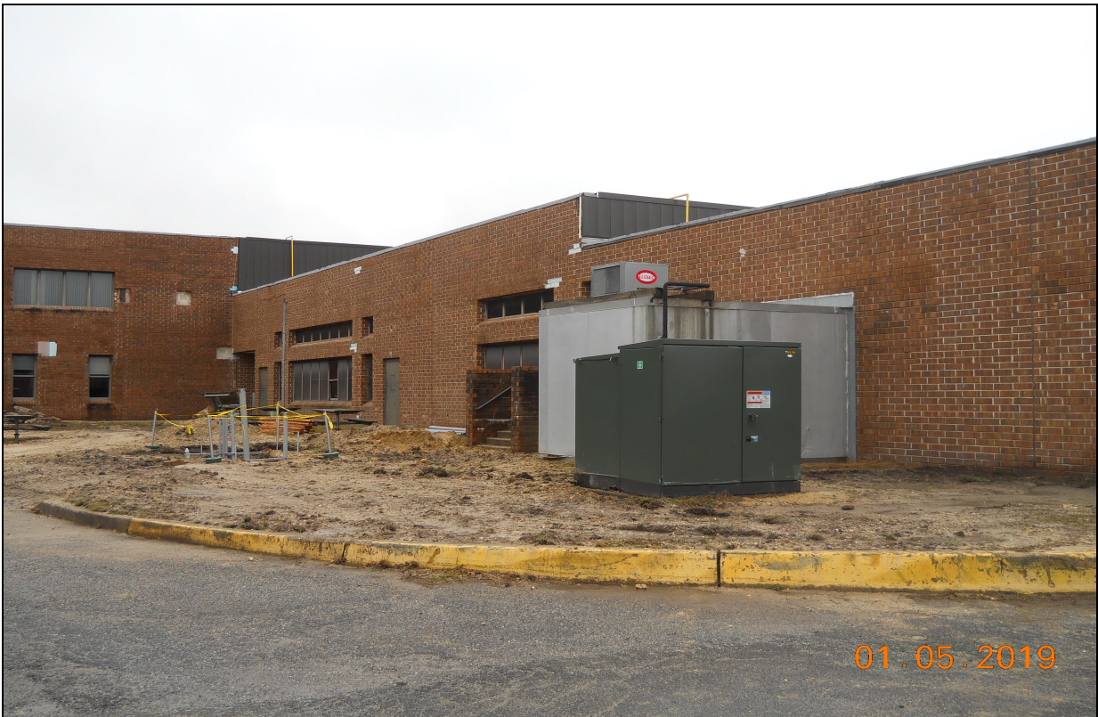
Pinelands Regional Sr. High School 6 New Emergency Generator Preparation
