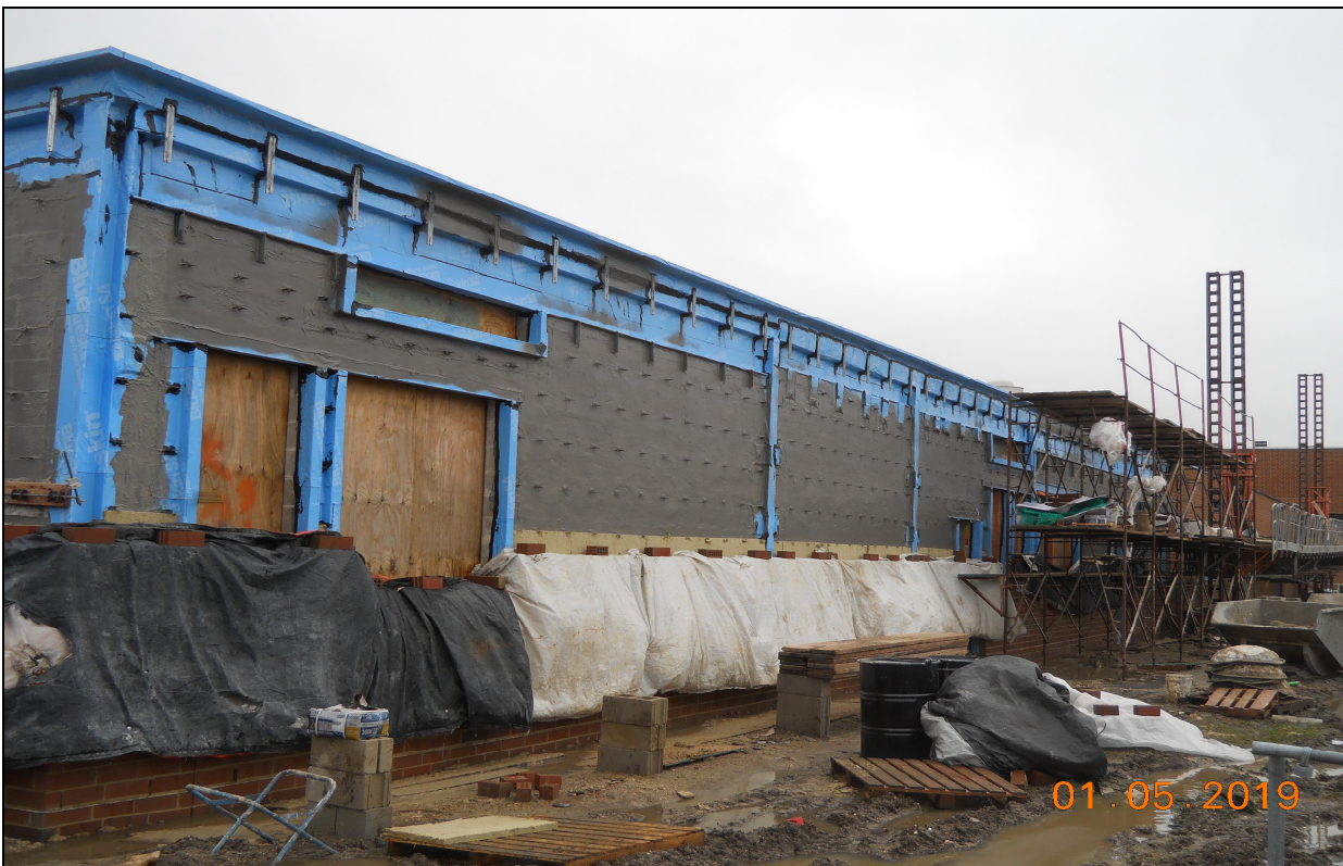
Pinelands Regional Sr. High School 6 Exterior Masonry Waterproofing (D-Wing North)
