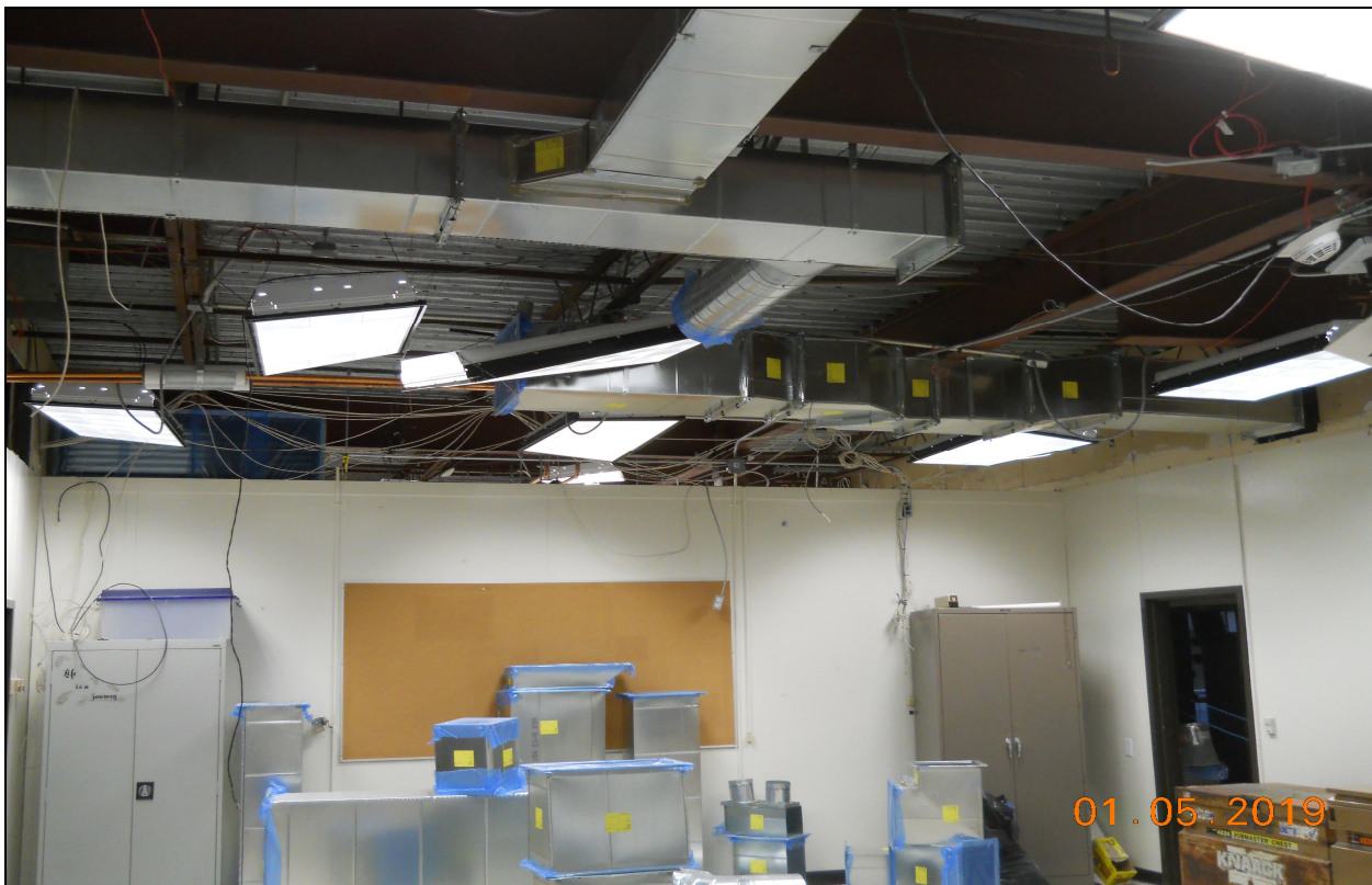
Pinelands Regional Sr. High School 6 3 rd Floor (A-Block) Classroom HVAC Ductwork
