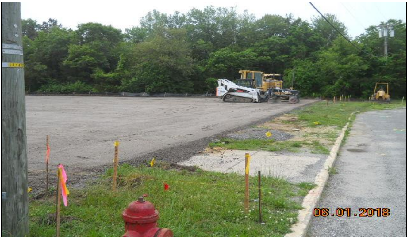
Pinelands Regional Tennis Courts – Subgrade Installation & Survey Layout
