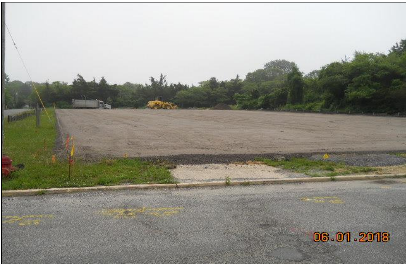
Pinelands Regional Tennis Courts – Subgrade Installation & Survey Layout
