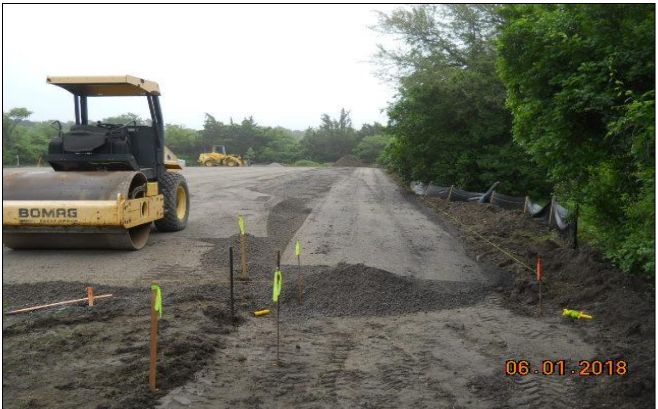
Pinelands Regional Jr. High – Subgrade Installation & Survey Layout
