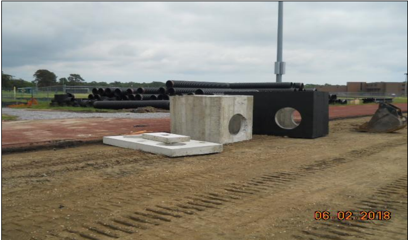
Pinelands Regional Athletic Field – Drainage System Structures
