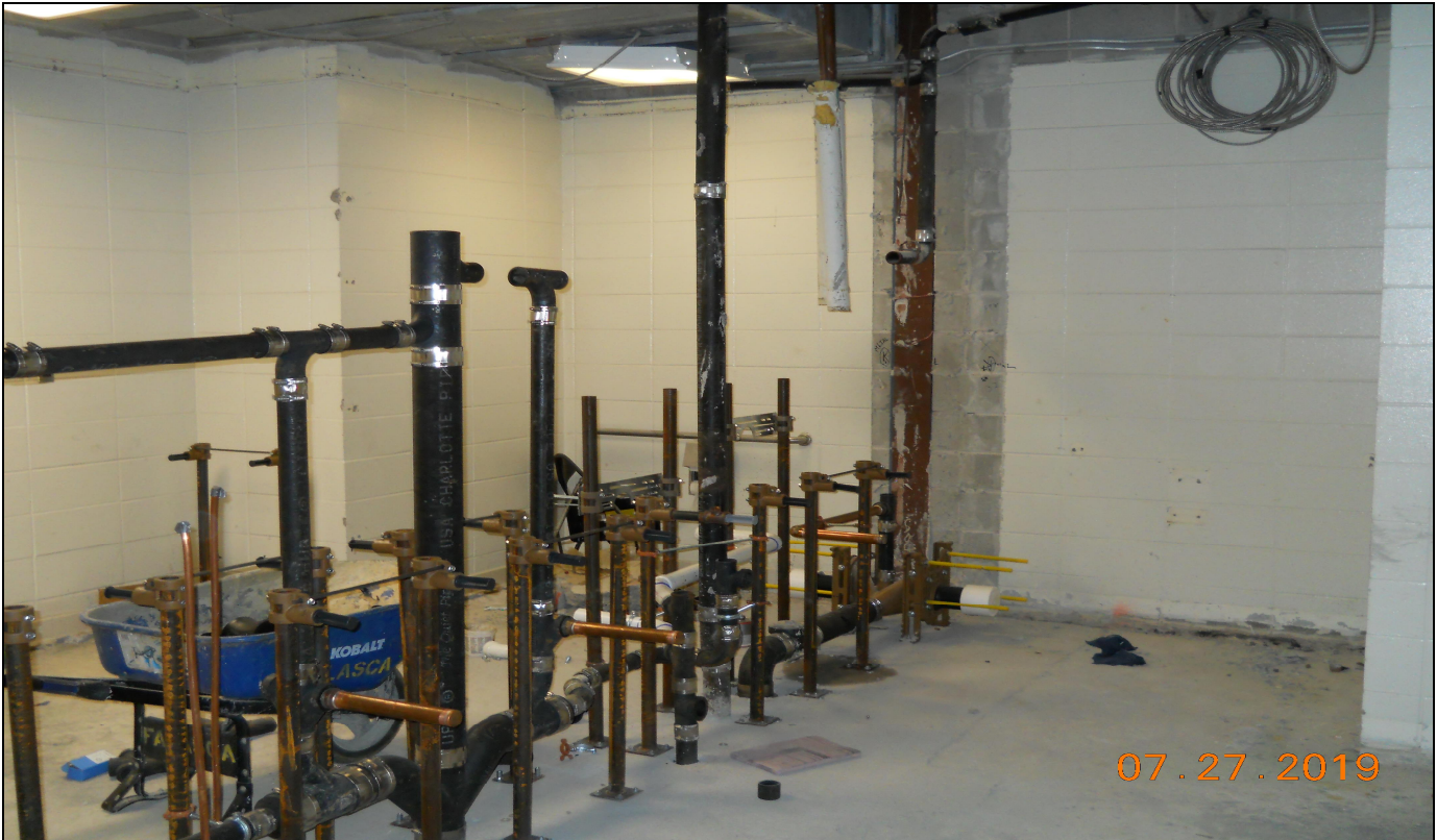
Pinelands Regional Jr. High School 6 Plumbing Rough-in (Locker-Room Bathrooms)
