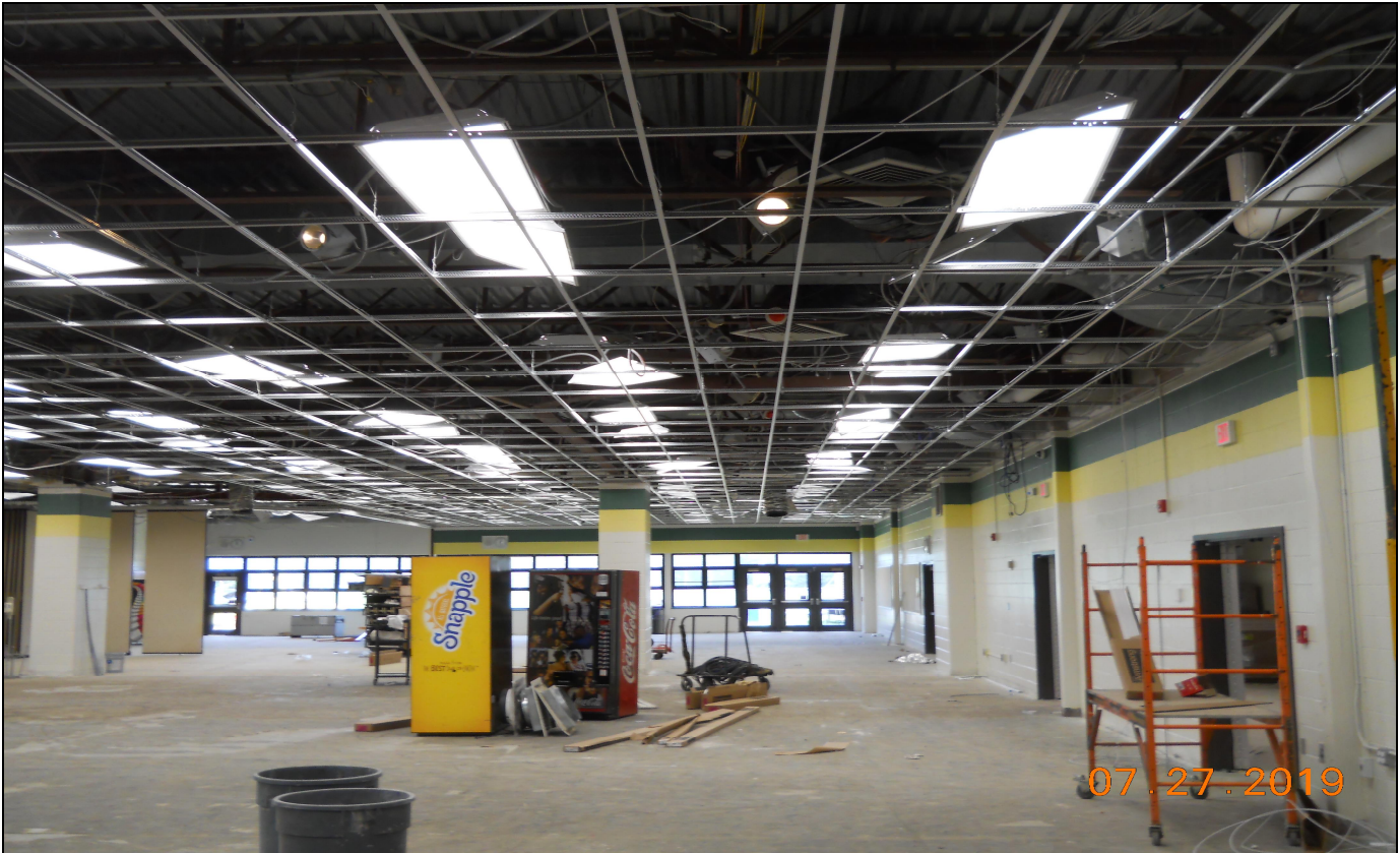
Pinelands Regional Jr. High School 6 Cafeteria Ceiling System Installation
