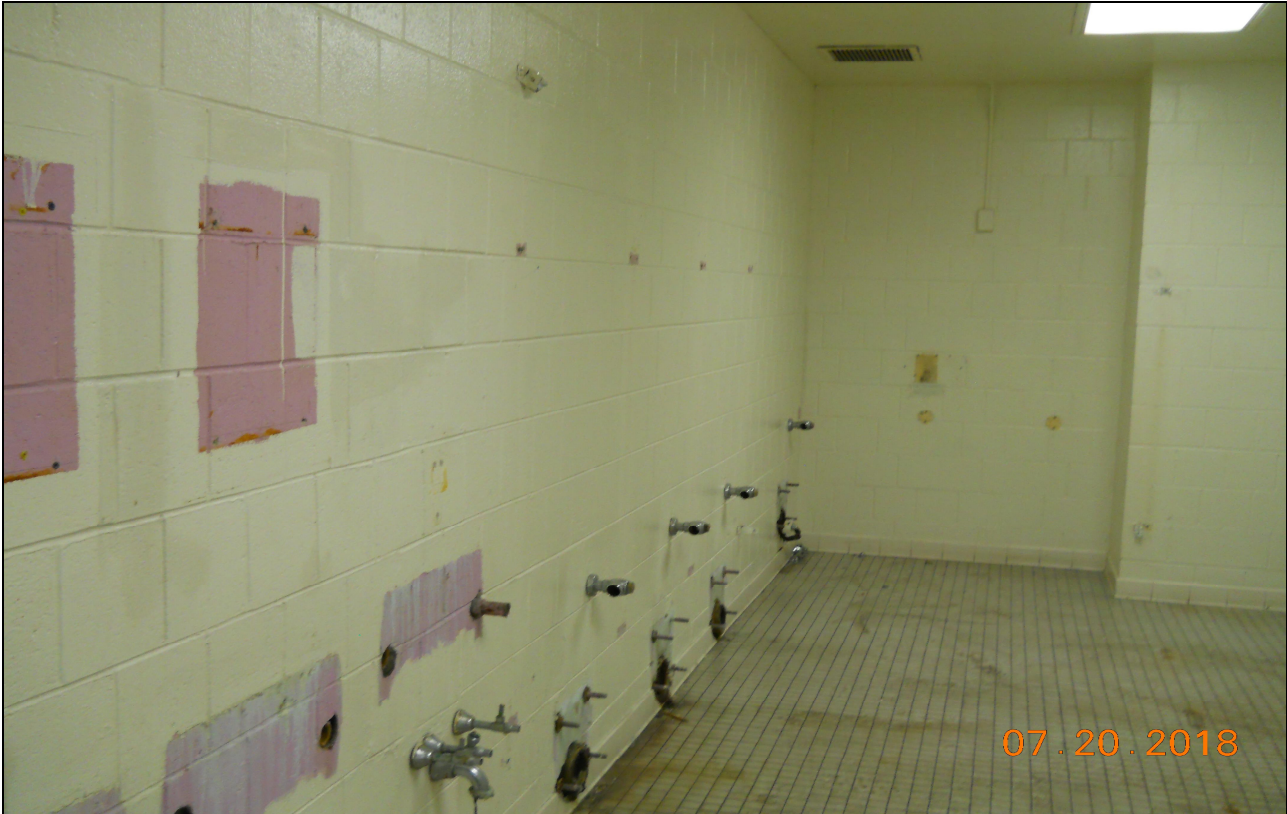
Pinelands Regional Sr. High School ó Removal of Bathroom Fixtures
