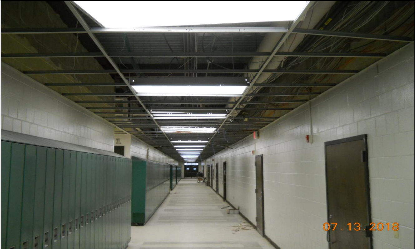
Pinelands Regional Sr. High School – Corridor Ceiling Tile Removal
