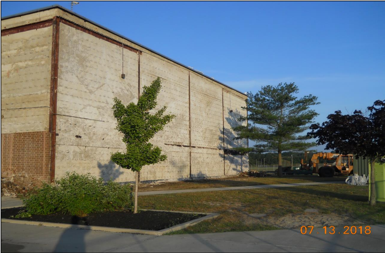
Pinelands Regional Sr. High School – Exterior Brick Fascia Removal
