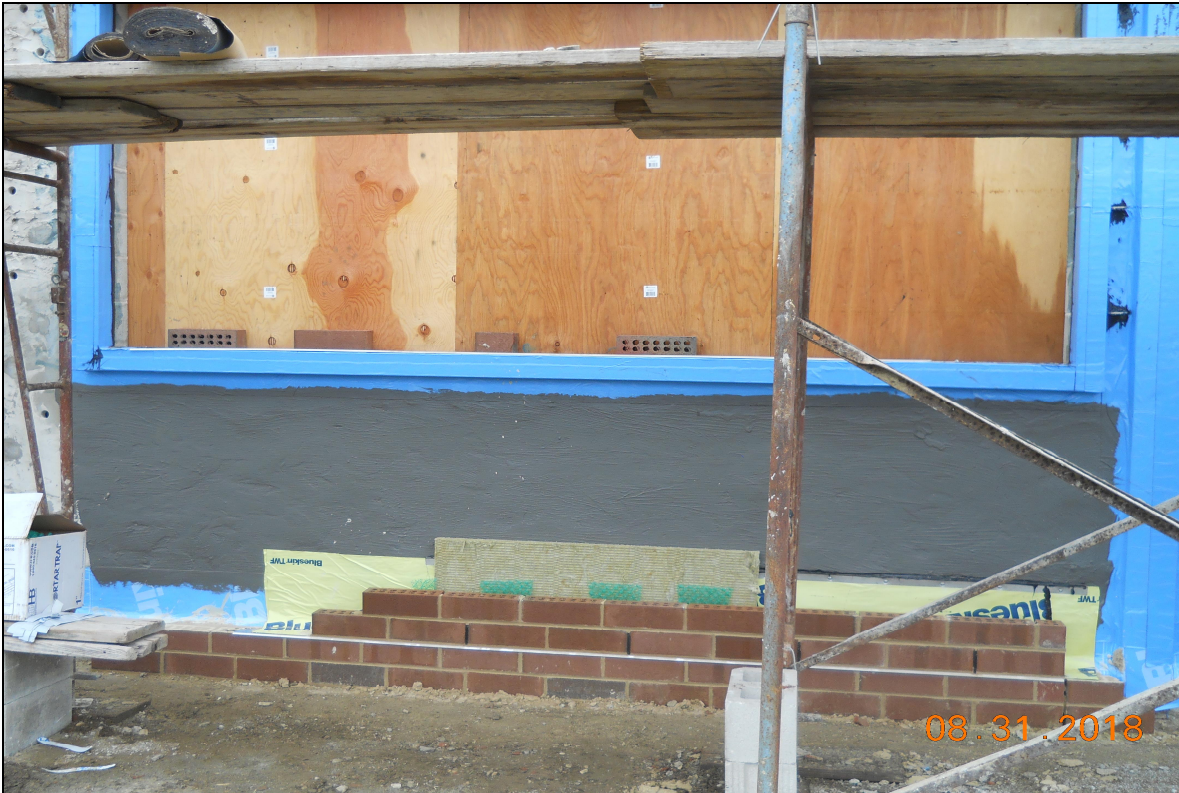
Pinelands Regional Sr. High School 6 Exterior Masonry Mock-up
