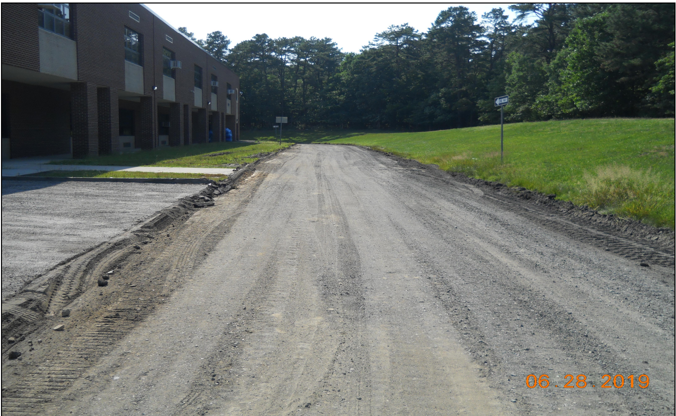
Pinelands Regional Jr. High School 6 Removal of Rear Roadway Asphalt
