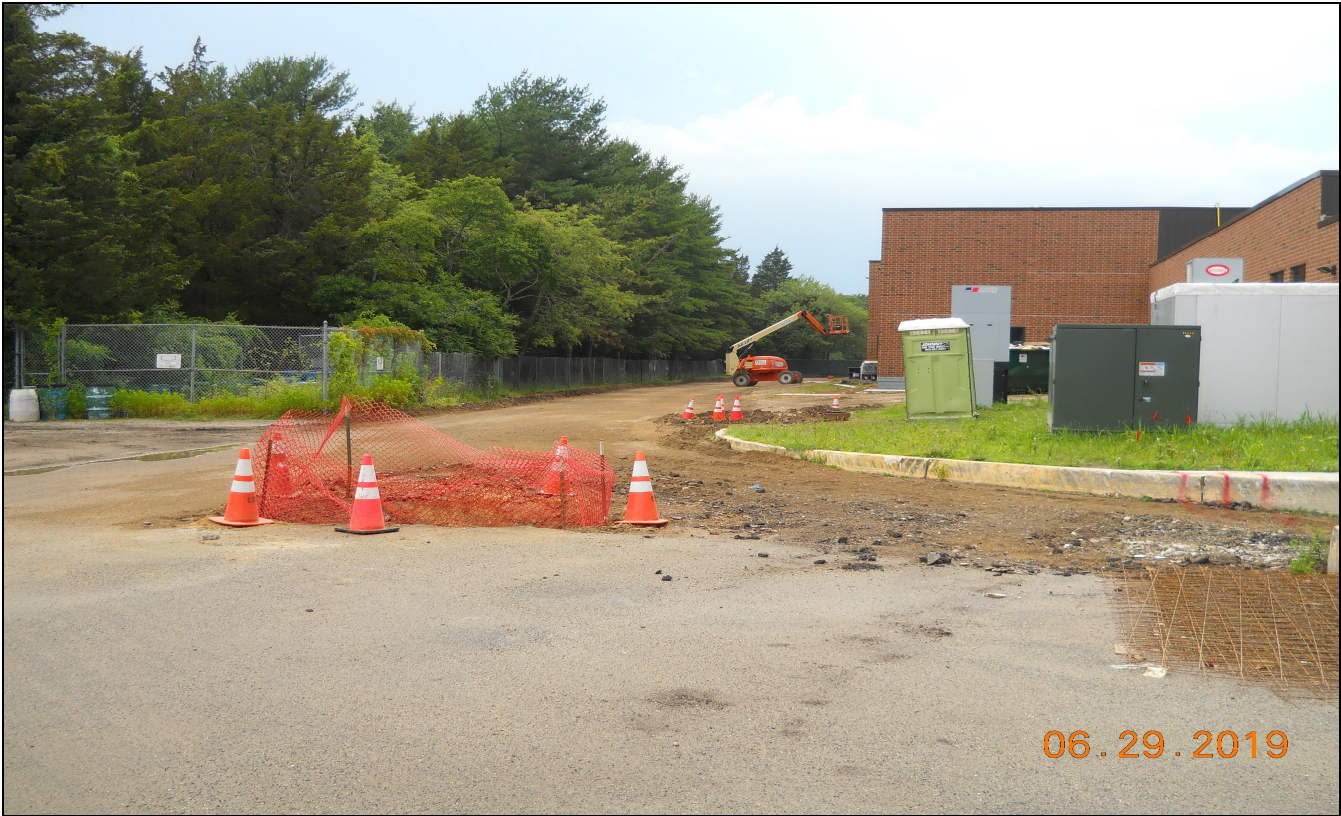
Pinelands Regional Sr. High School 6 Storm-water & Rear Roadway Asphalt Removal
