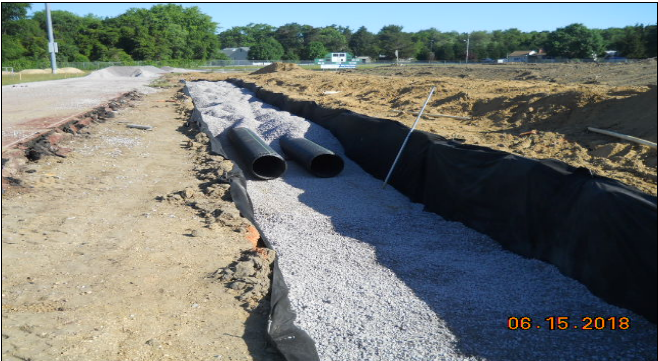
Pinelands Regional Athletic Field – Drainage System Installation
