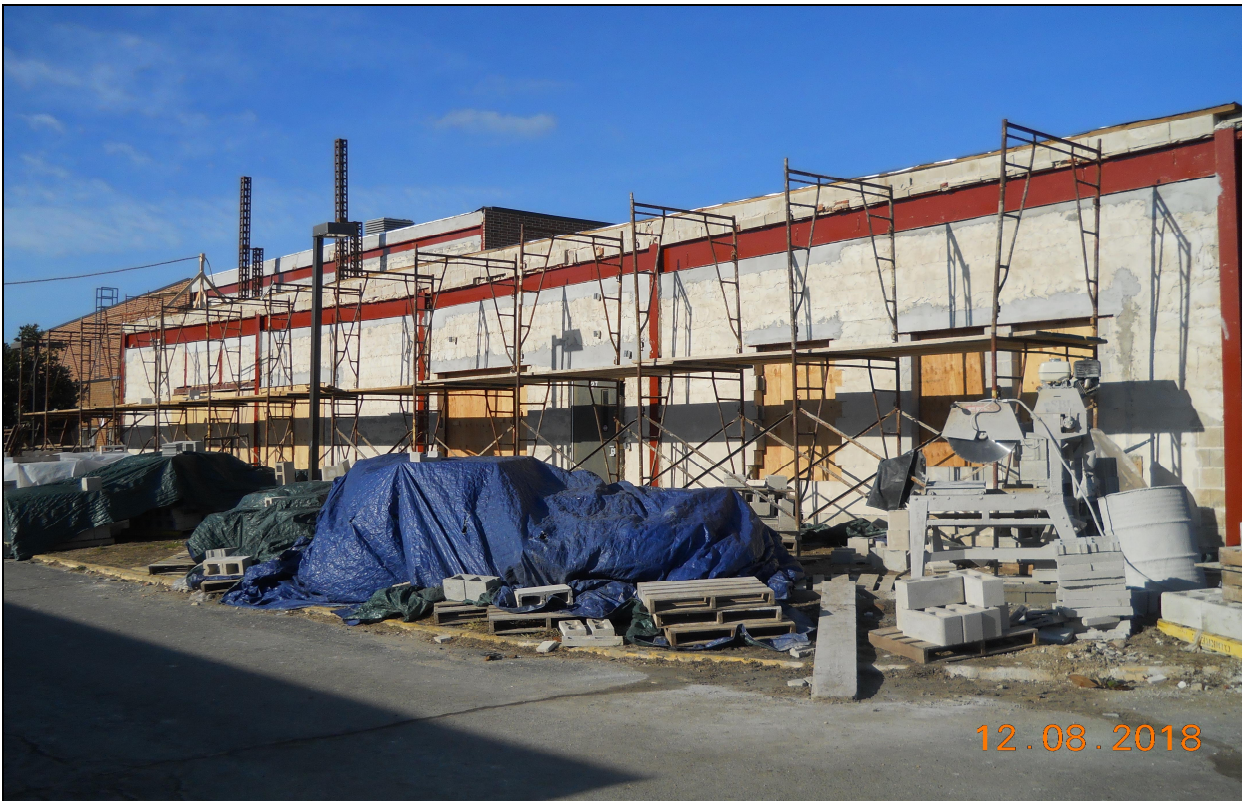
Pinelands Regional Sr. High School ó Exterior Masonry Waterproofing / Brick Veneer Installation
