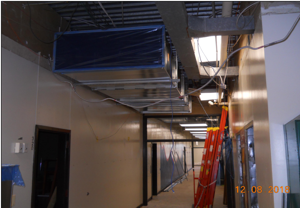
Pinelands Regional Sr. High School 6 HVAC Ductwork Installation (3 rd Floor Corridor)
