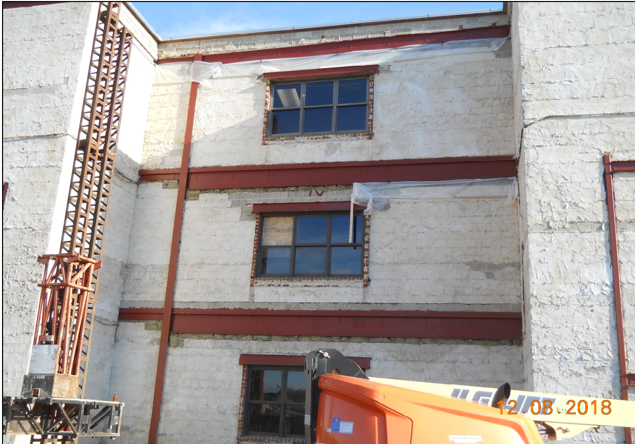
Pinelands Regional Sr. High School 6 Exterior Masonry Preparation (A-Wing West)
