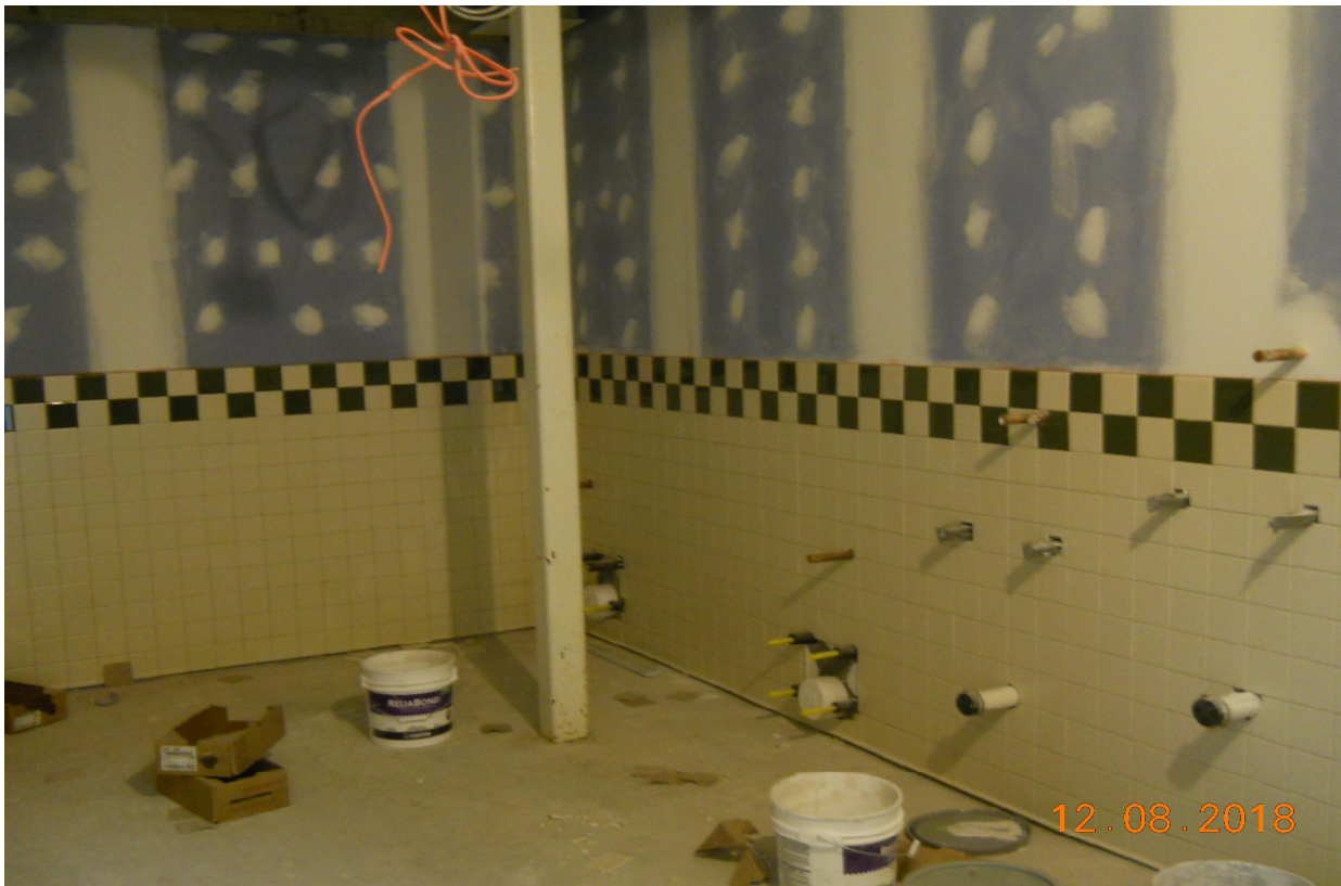
Pinelands Regional Sr. High School ó Bathroom Ceramic Tile Installation (1 st Floor)
