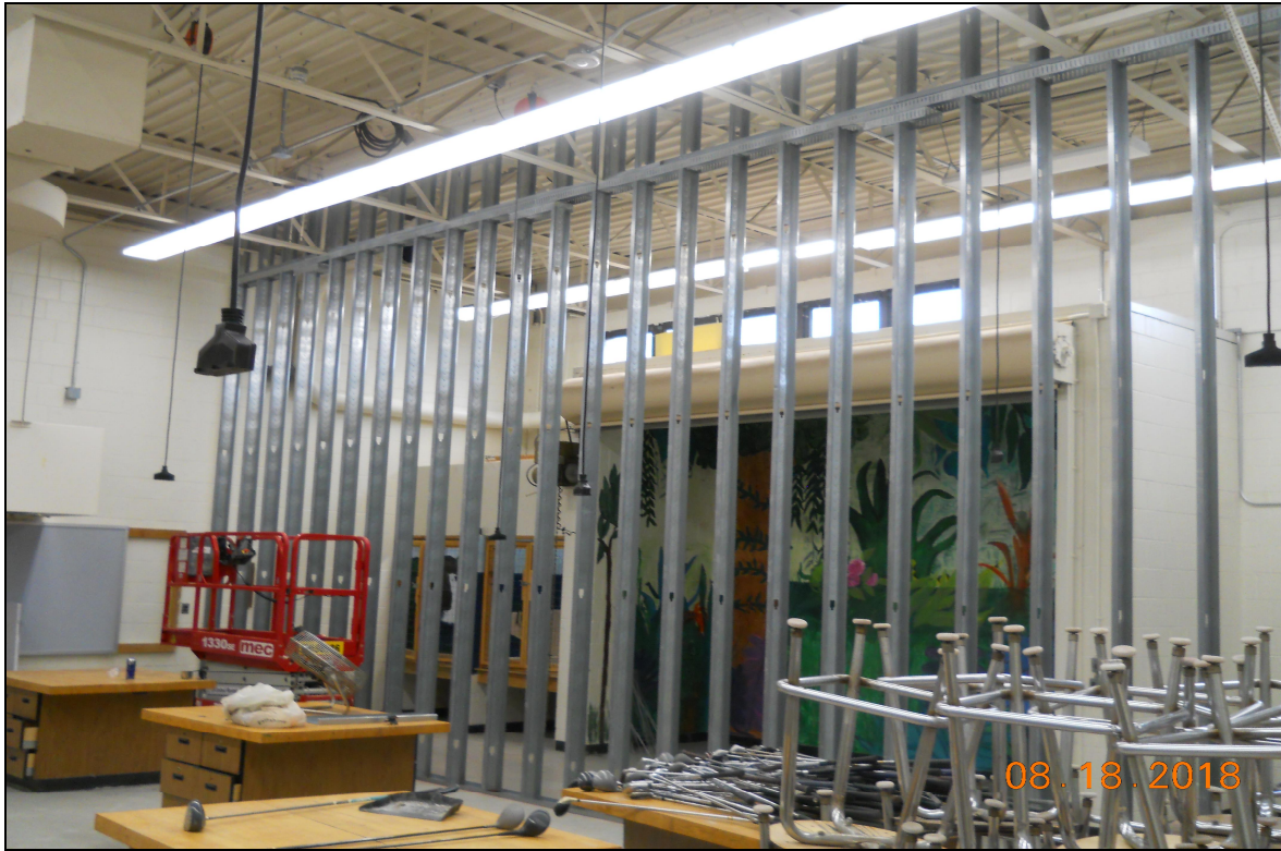
Pinelands Regional Sr. High School 6 Temporary Wall Installation
