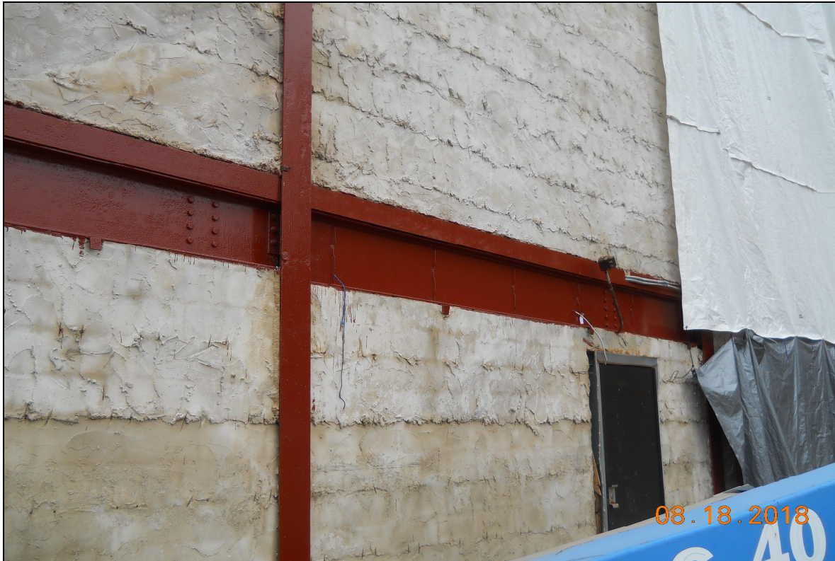
Pinelands Regional Sr. High School 6 Structural Steel (Cleaned / Painted)
