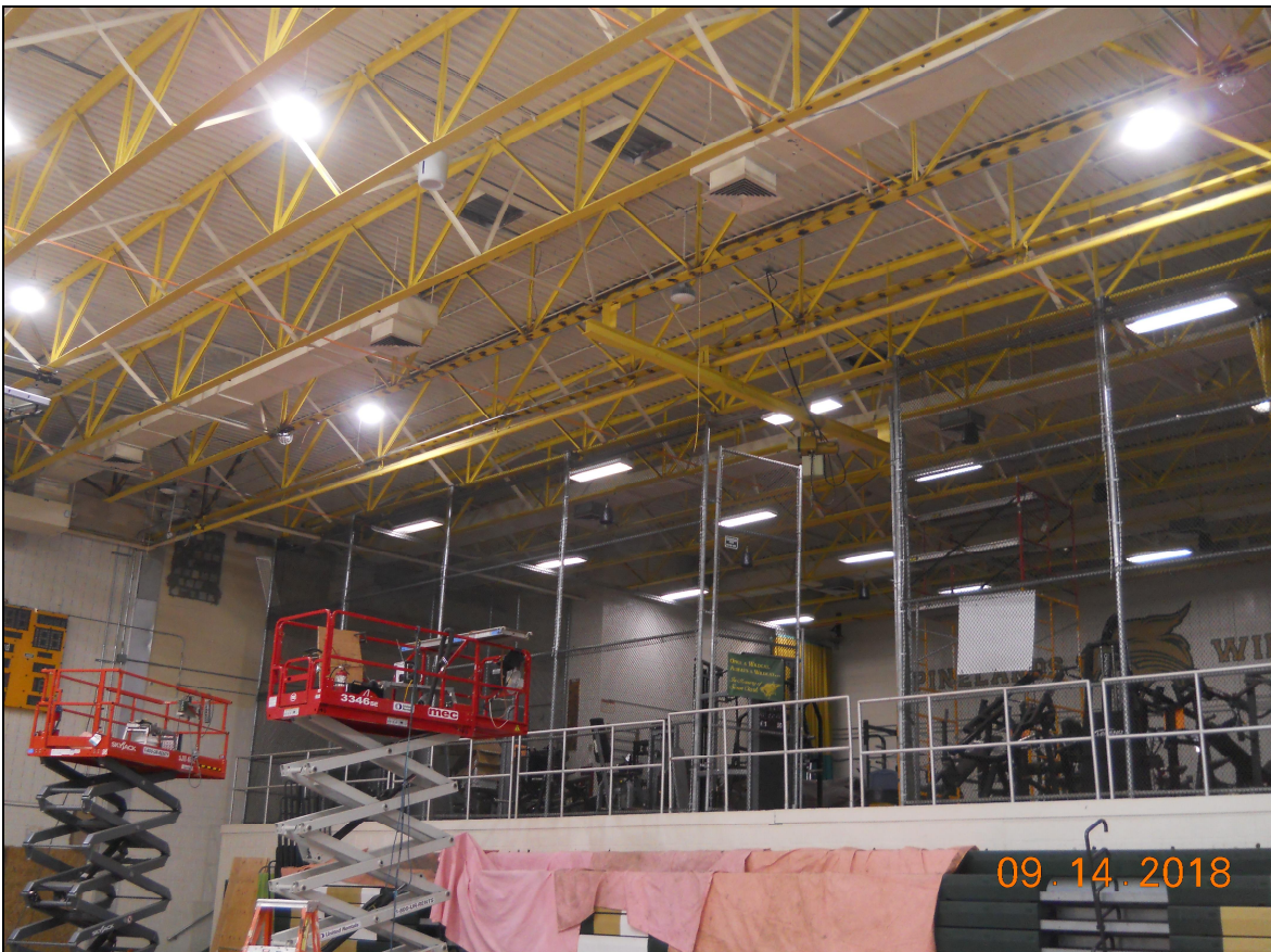
Pinelands Regional Sr. High School 6 Gym Structure Modification (New HVAC Units)
