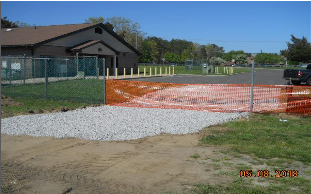
Pinelands Regional Athletic Field 6 Soil Erosion Traffic pad
