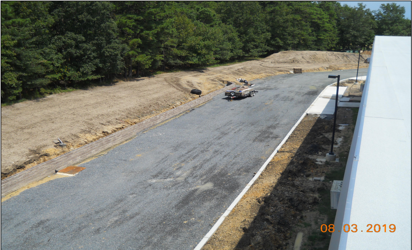
Pinelands Regional Sr. High School 6 Rear Service Road- Sidewalk & Curbing Installation
