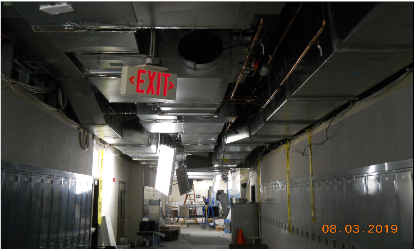
Pinelands Regional Jr. High School 6 Corridor Ductwork Installation (2 nd Floor)
