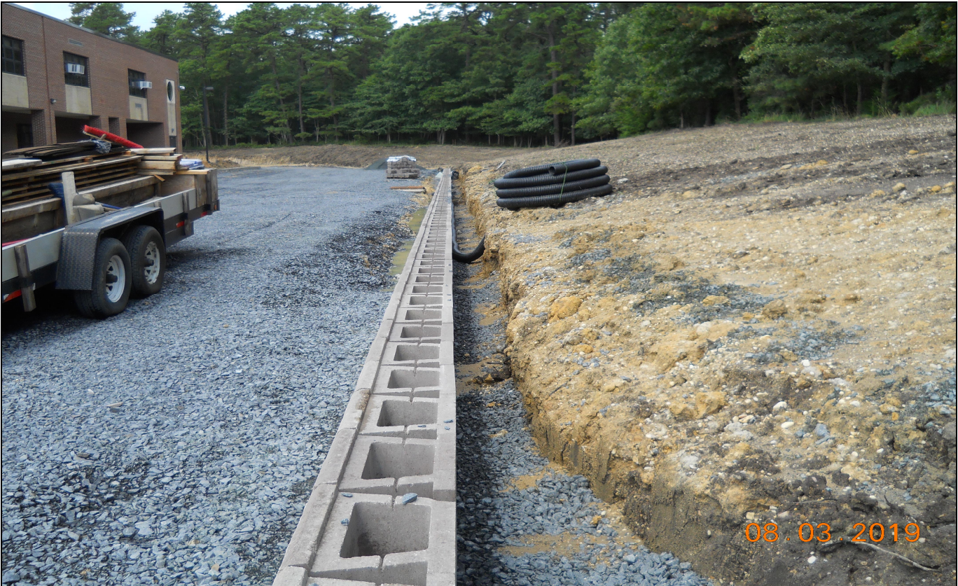
Pinelands Regional Jr. High School 6 Site Preparation Rear Bus Lane (Retaining Wall)
