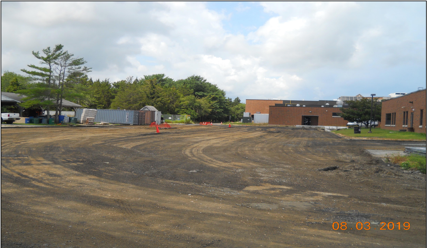
Pinelands Regional Sr. High School 6 Rear Parking Lot Asphalt Milling / Removal
