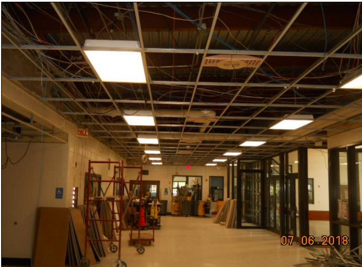
Pinelands Regional Sr. High School 6 Corridor Ceiling Tile Removal
