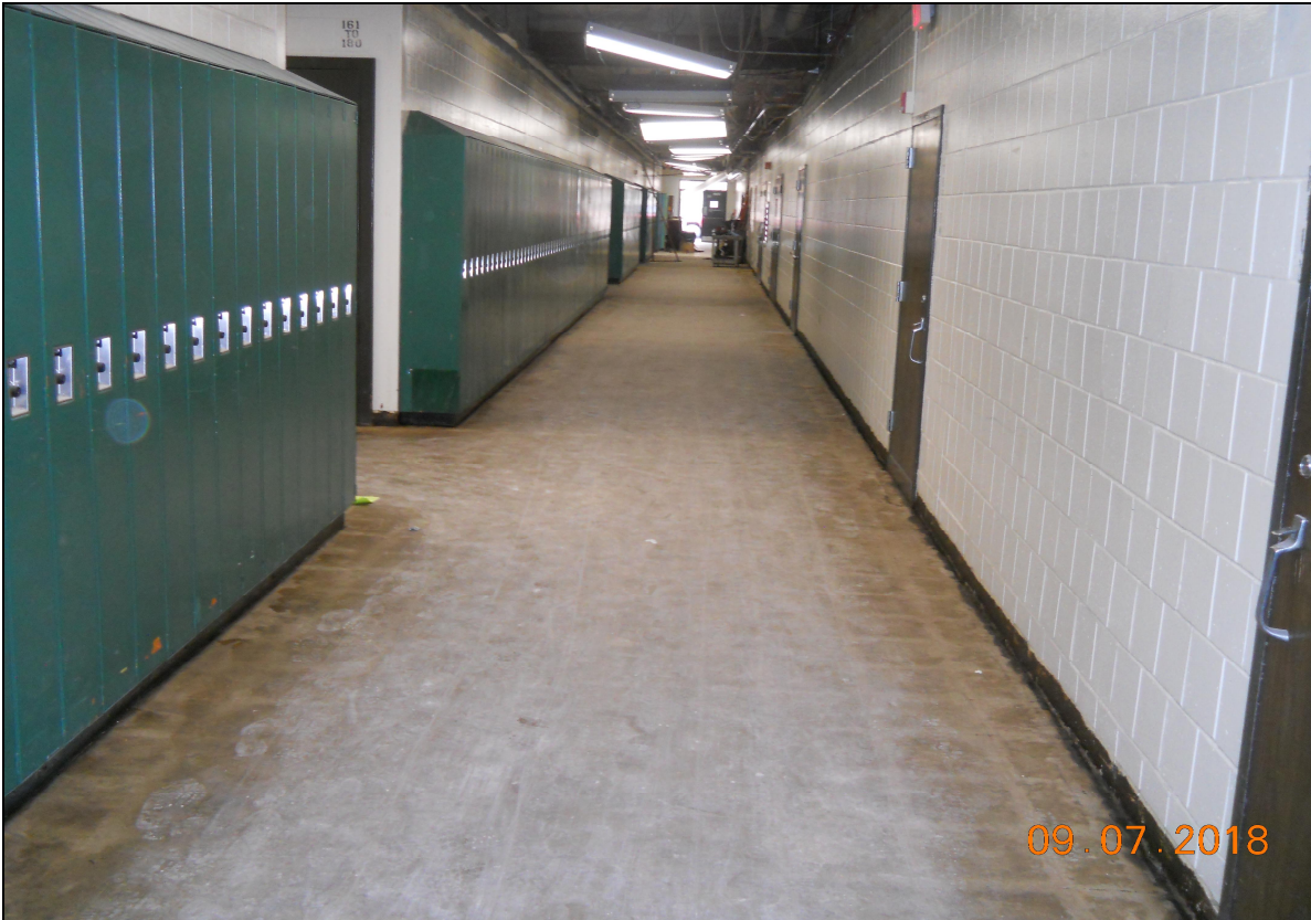
Pinelands Regional Sr. High School 6 Removal of Corridor Floor Tile (D Wing)
