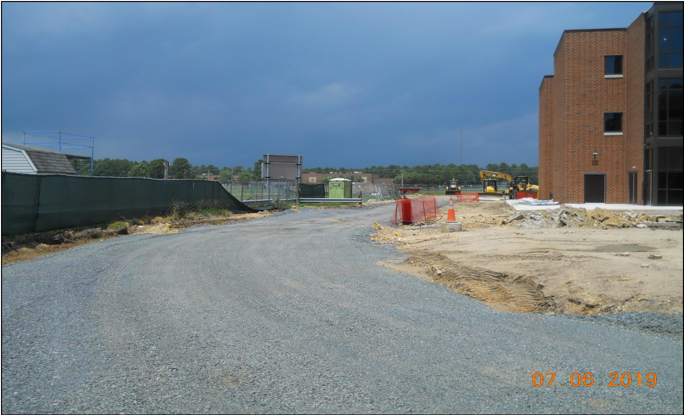
Pinelands Regional Sr. High School 6 Gravel Base Installation (Rear Service Road)
