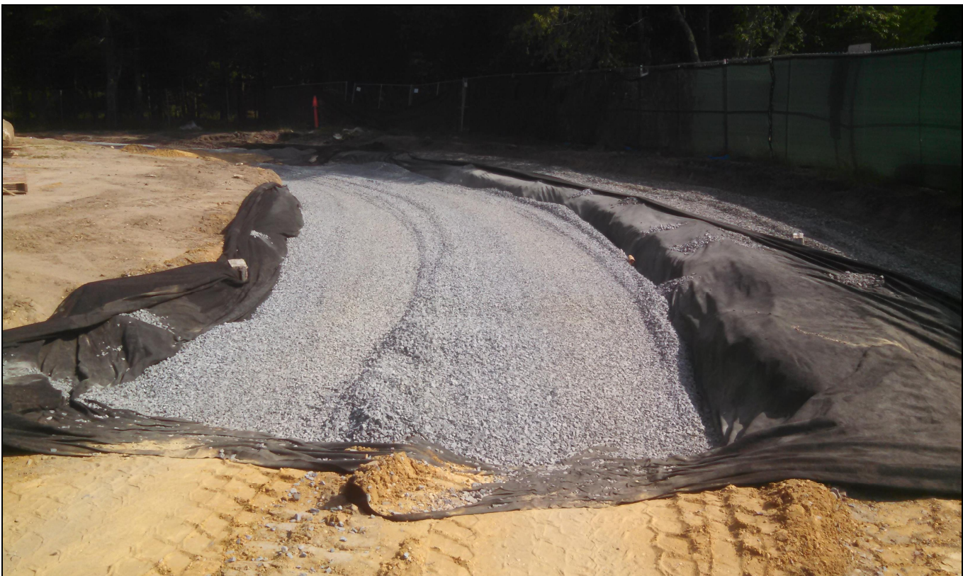
Pinelands Regional Sr. High School 6 Rear Service Road Subgrade Installation
