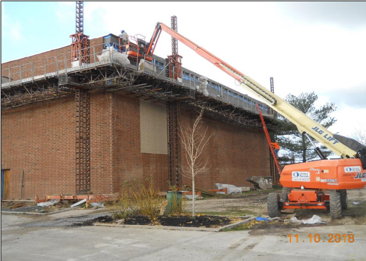
Pinelands Regional Sr. High School □ Exterior Masonry Waterproofing / Brick Veneer Installation
