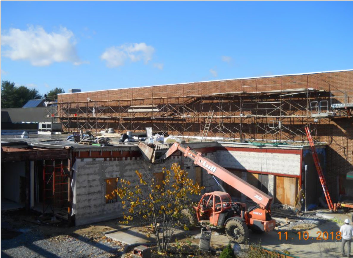
Pinelands Regional Sr. High School □ Exterior Masonry Waterproofing / Brick Veneer Installation
