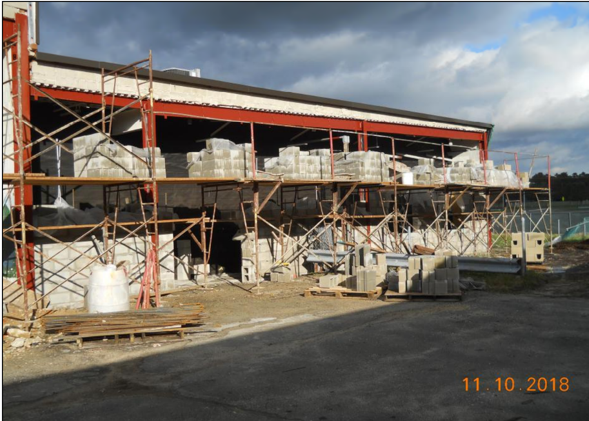
Pinelands Regional Sr. High School □ Exterior Masonry Wall Installation D-Wing East
