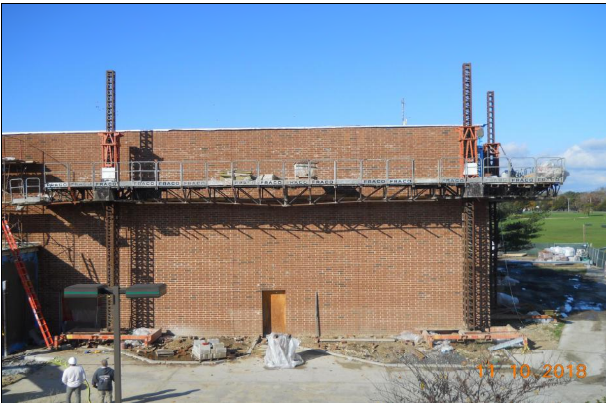
Pinelands Regional Sr. High School □ Exterior Masonry Waterproofing / Brick Veneer Installation
