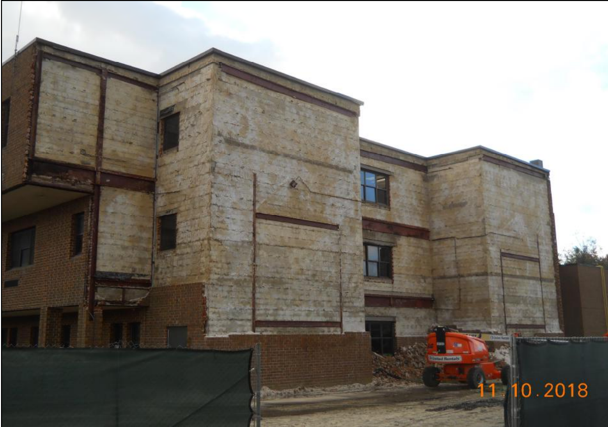
Pinelands Regional Sr. High School □ Exterior Masonry Facia Demolition A-Wing West
