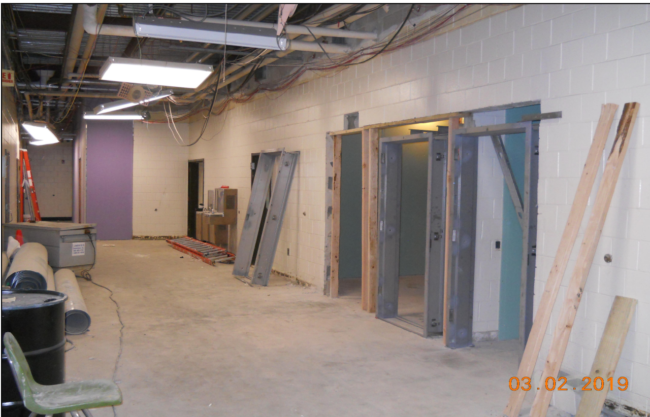
Pinelands Regional Sr. High School ó Installation of Bathroom Door Frames (Block B)
