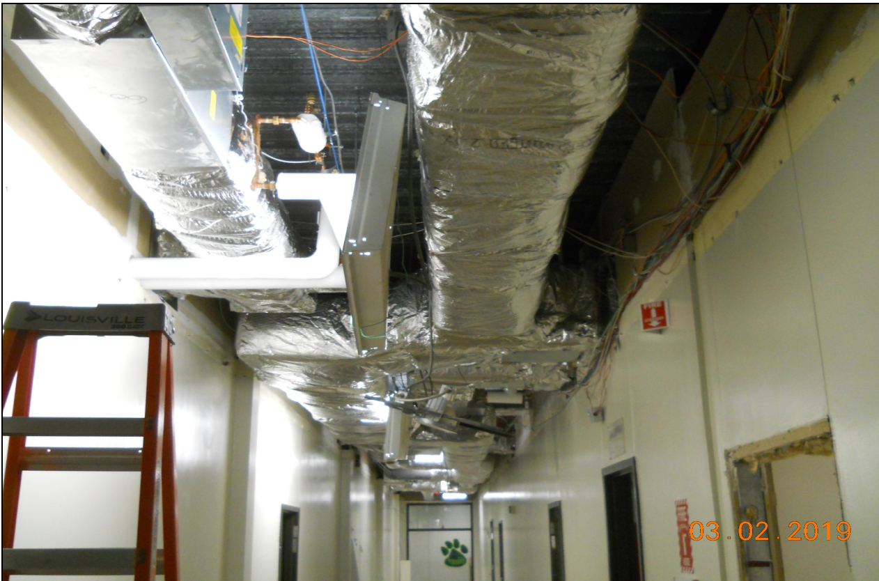
Pinelands Regional Sr. High School 6 HVAC Ductwork Insulation
