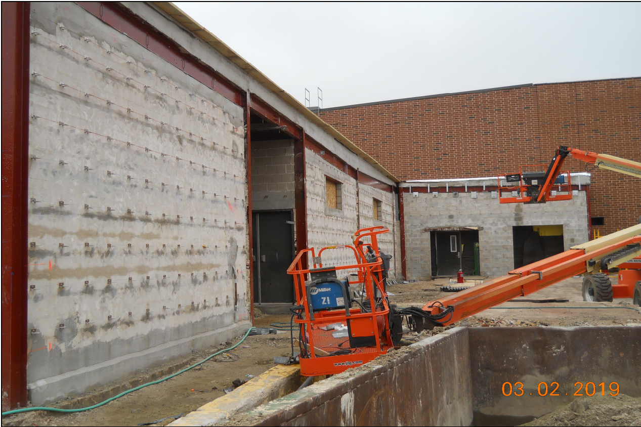
Pinelands Regional Sr. High School 6 Exterior Masonry Reconstruction & Preparation (Block C East)
