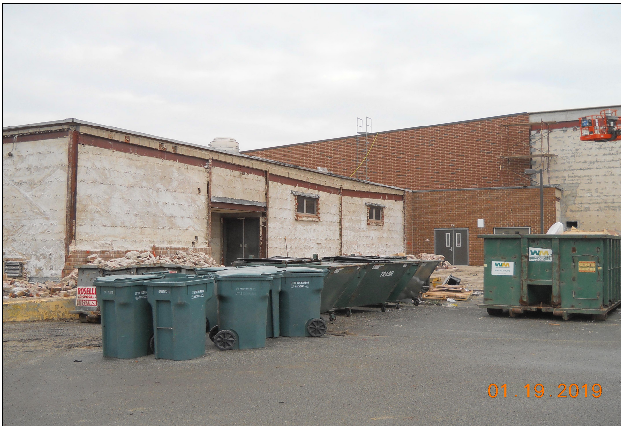
Pinelands Regional Sr. High School 6 Exterior Masonry Facia Removal (Kitchen East)
