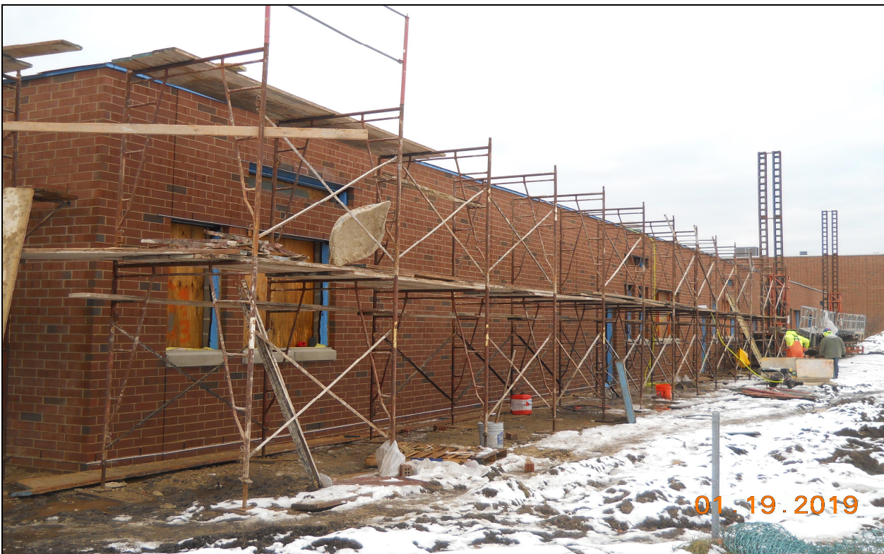
Pinelands Regional Sr. High School 6 Exterior Masonry Installation (D-Wing North)
