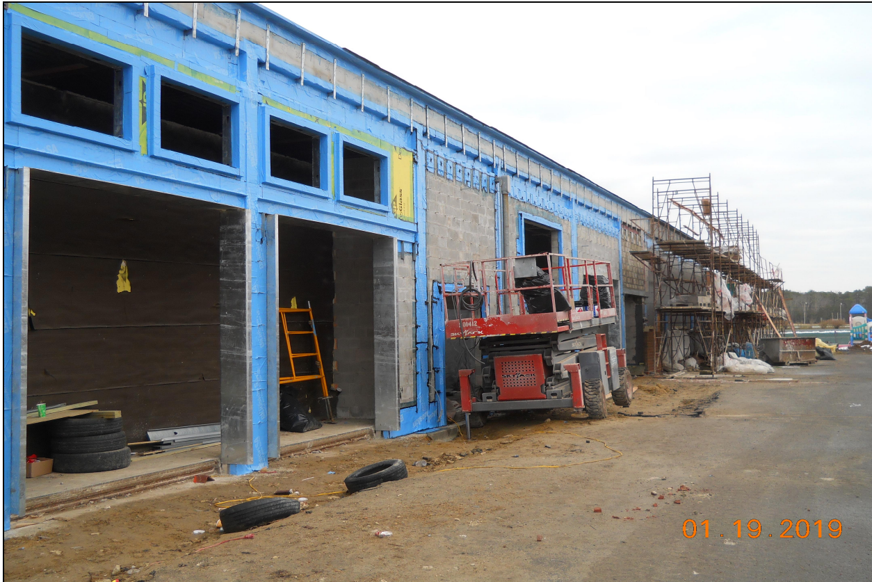
Pinelands Regional Sr. High School 6 Exterior Masonry Installation (D-Wing East)
