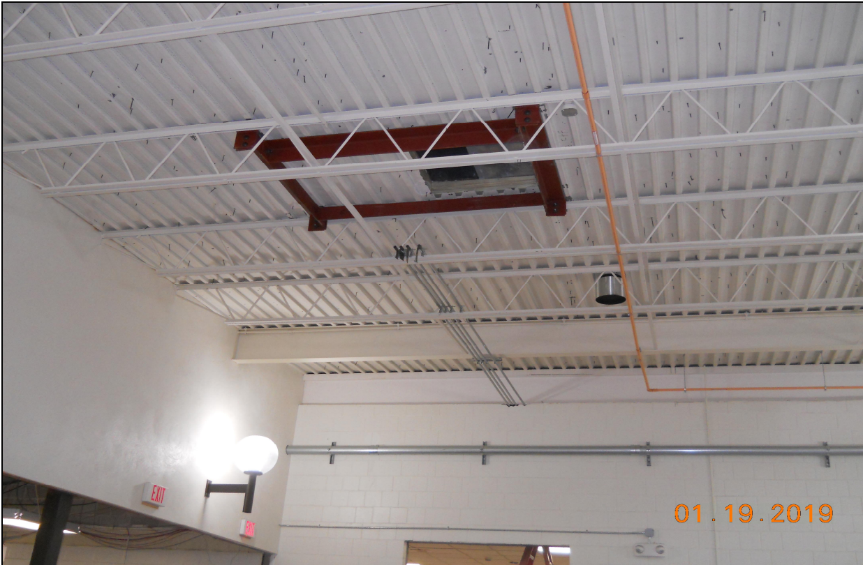
Pinelands Regional Sr. High School 6 Atrium Roof Structure Modification (HVAC Unit)
