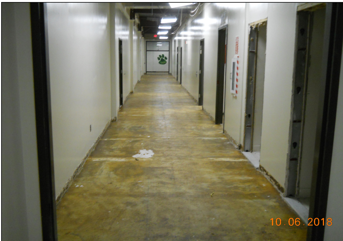
Pinelands Regional Sr. High School 6 Corridor Floor Tile Removal -Block A North-
