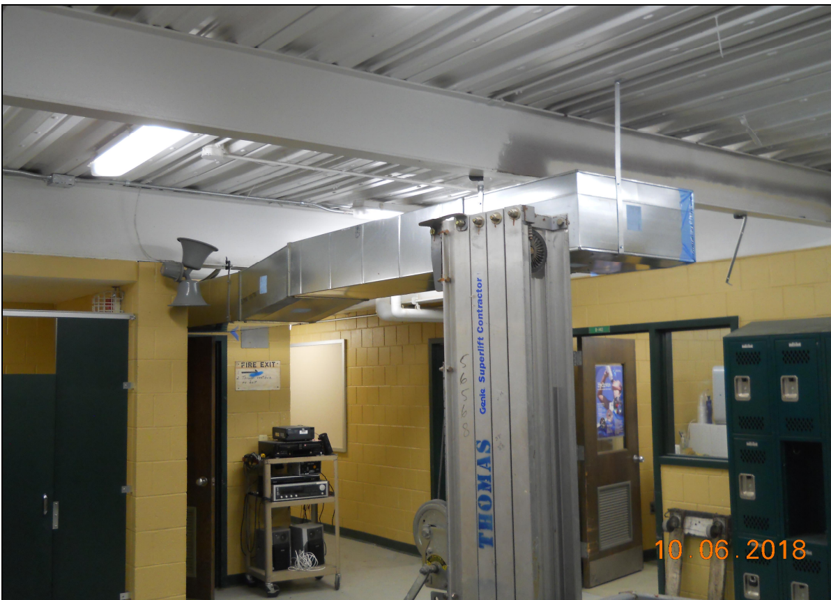
Pinelands Regional Sr. High School 6 Locker Room HVAC Ductwork Installation
