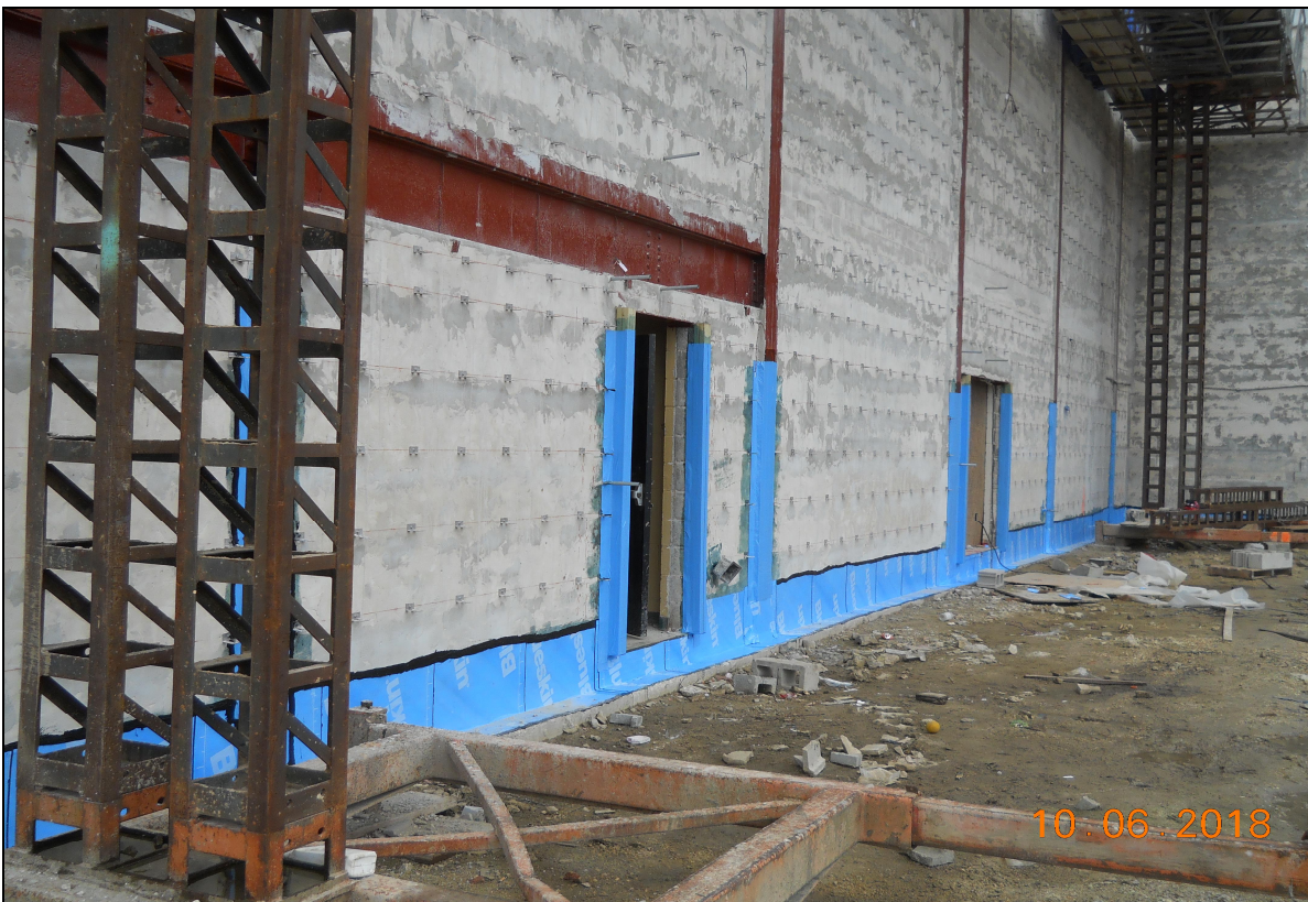
Pinelands Regional Sr. High School 6 Exterior Masonry Waterproofing
