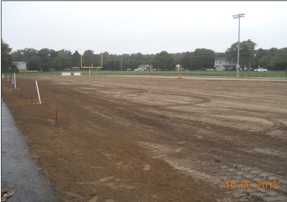
Pinelands Regional Athletic Field 6 Final Grading For Sod Turf Installation
