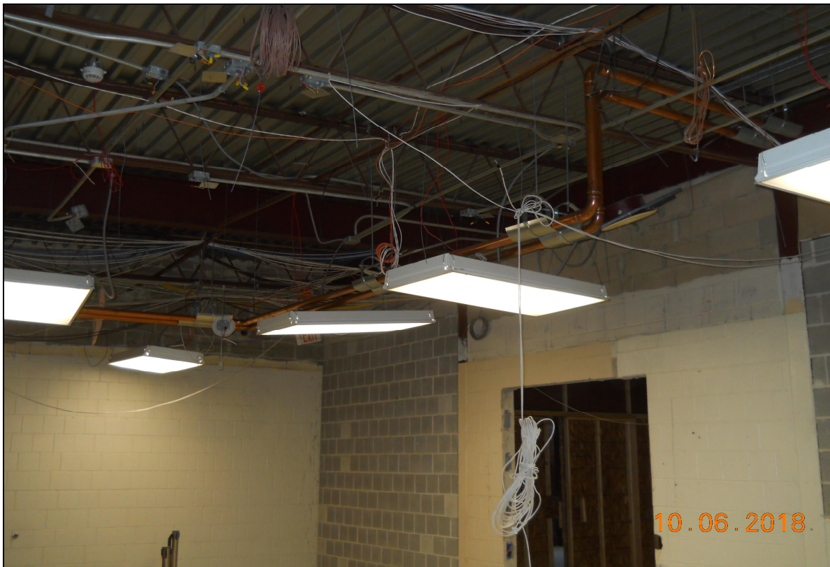
Pinelands Regional Sr. High School 6 HVAC Heating Piping Rough-in
