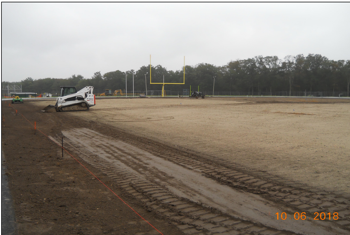
Pinelands Regional Athletic Field 6 Final Grading For Sod Turf Installation
