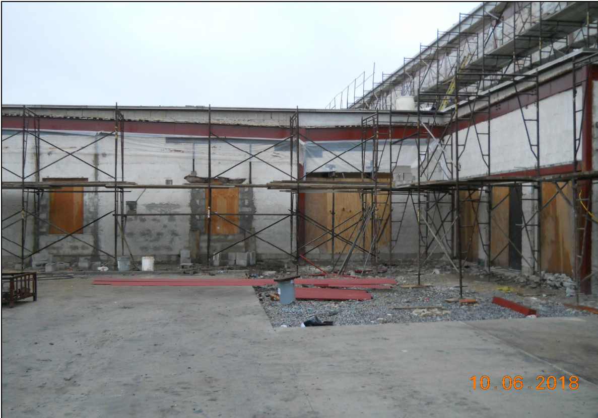
Pinelands Regional Sr. High School 6 Exterior Masonry Window Modifications
