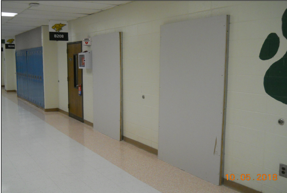
Pinelands Regional Jr. High School 6 Construction Safety Barricade (Bathroom Renovation 2 nd Floor)
