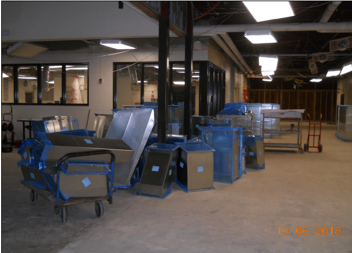
Pinelands Regional Sr. High School 6 Main Office HVAC Ductwork (New)
