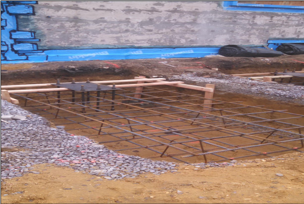
Pinelands Regional Sr. High School 6 New Entrance Canopy Foundation (Rebar)
