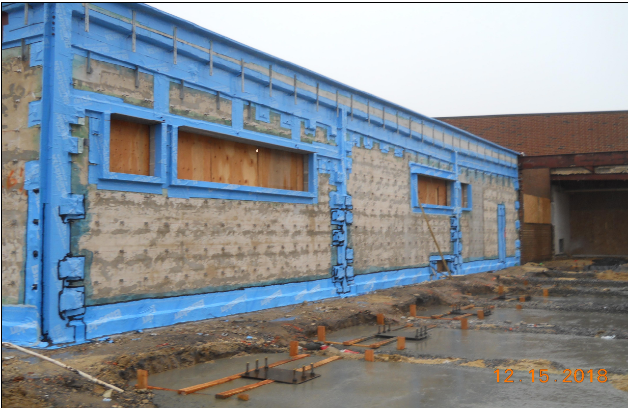
Pinelands Regional Sr. High School ó Exterior Masonry Waterproofing
