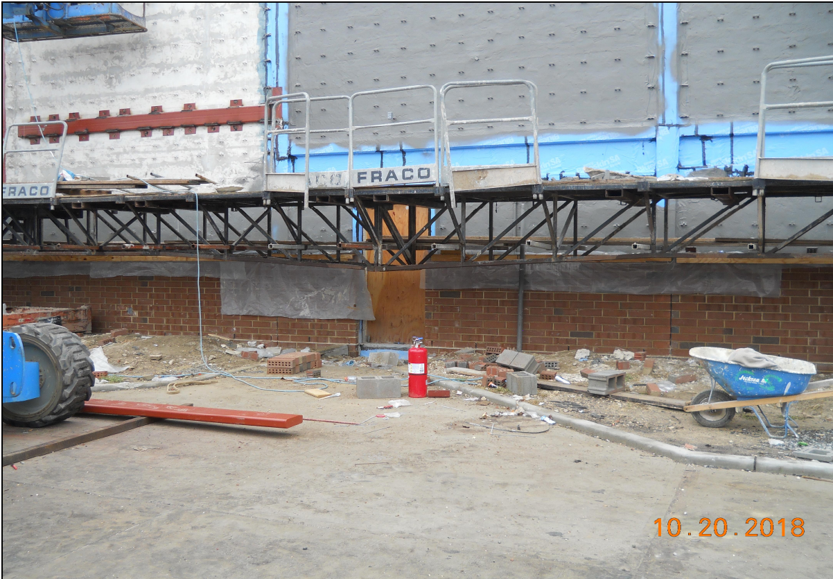
Pinelands Regional Sr. High School 6 Exterior Masonry Waterproofing / Brick Veneer Installation
