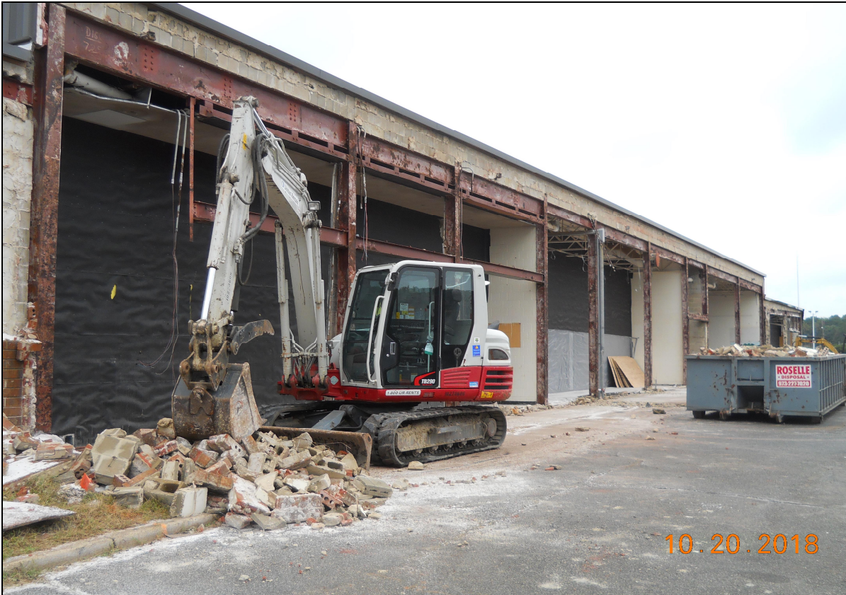
Pinelands Regional Sr. High School 6 Exterior Masonry Demolition > D-Wing East
