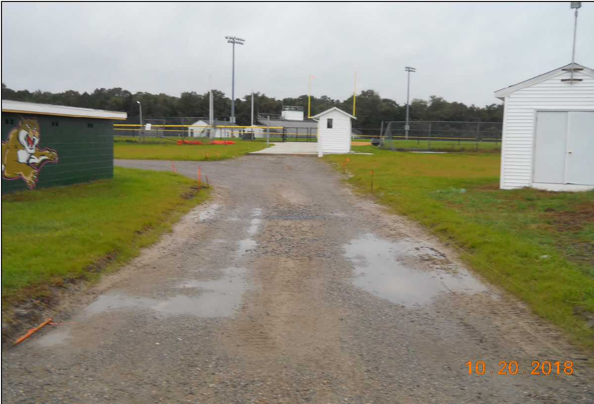
Pinelands Regional Athletic Field 6 Access Walkway Sub-base for Asphalt Paving
