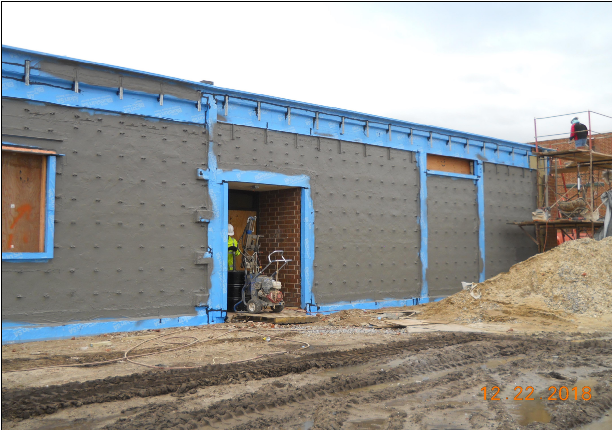
Pinelands Regional Sr. High School 6 Exterior Masonry Waterproofing (D-Wing North)
