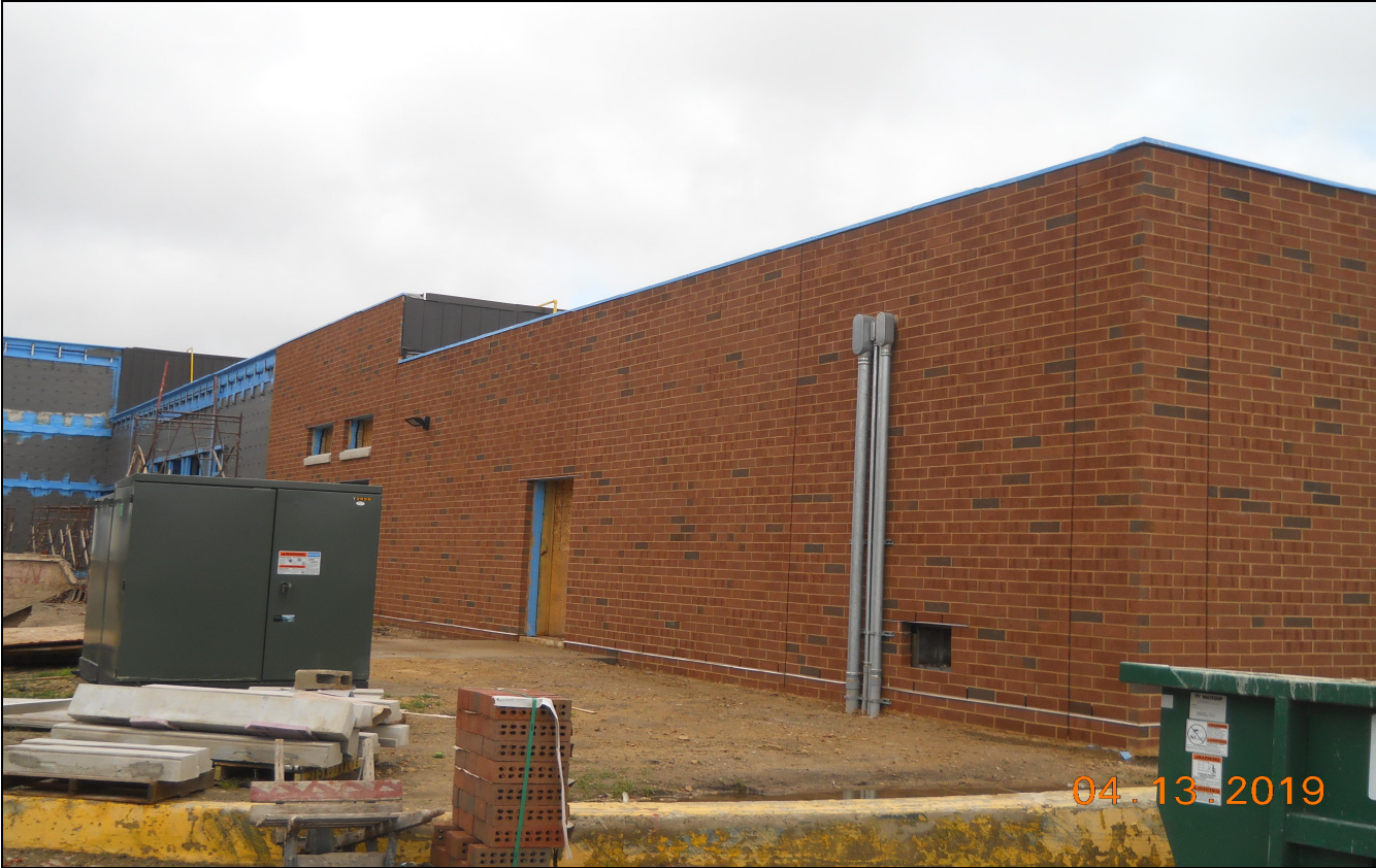
Pinelands Regional Sr. High School ó Exterior Brick- Installation (Block C South ó Cafeteria)
