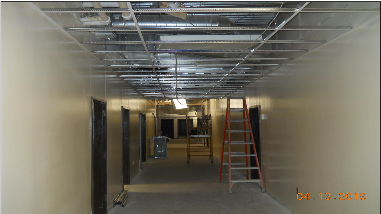
Pinelands Regional Sr. High School 6 Student Corridor Paint & Ceiling Grid (Block A 3 rd floor)
