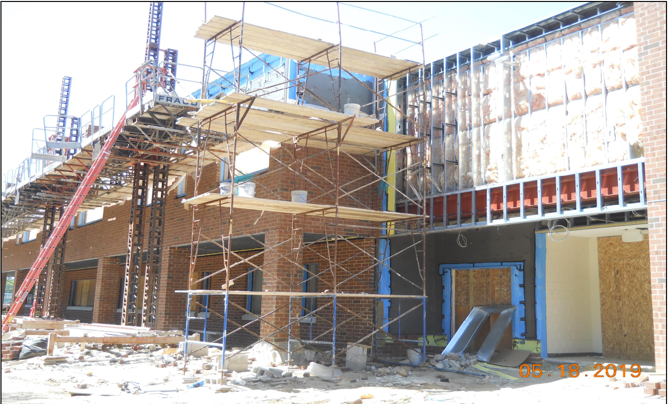
Pinelands Regional Sr. High School 6 Exterior Preparation & Brick Installation (Block A - South)
