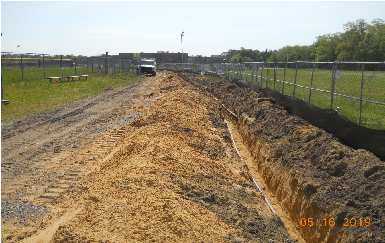
Pinelands Regional Sr. High School 6 Underground Electrical Piping (Walkway Lighting)
