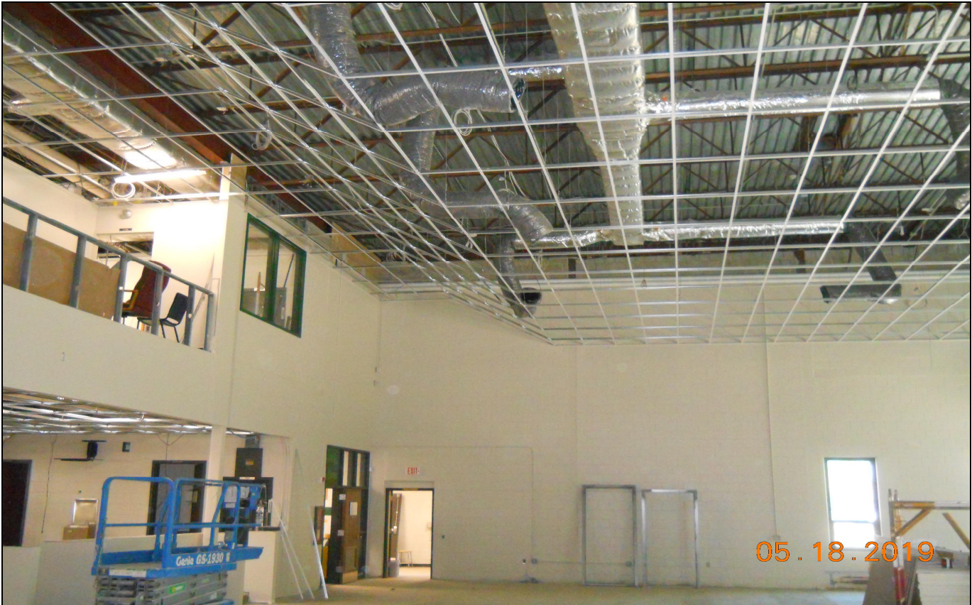
Pinelands Regional Sr. High School 6 Ceiling Installation Media Center (Block C)
