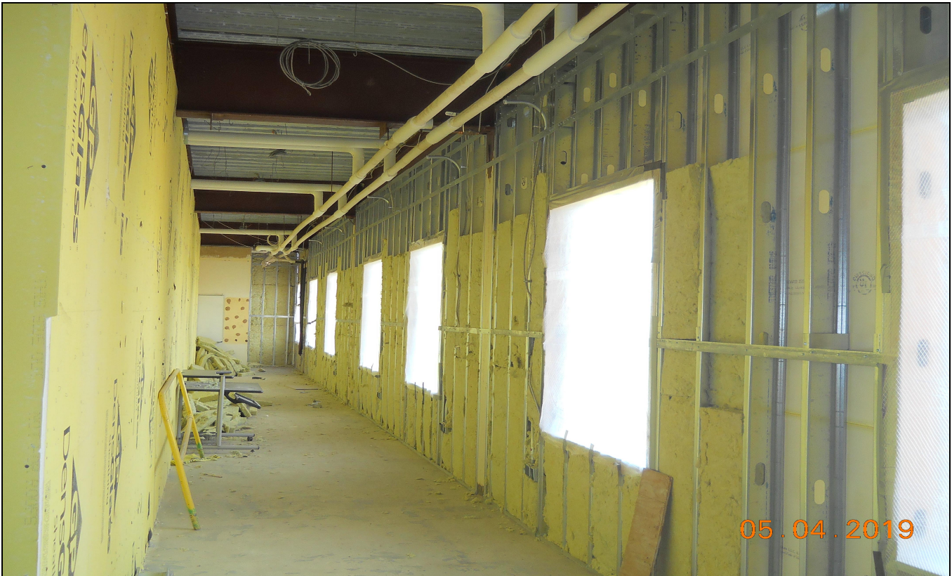
Pinelands Regional Sr. High School 6 Exterior Wall & Insulation Installation (Block A North)
