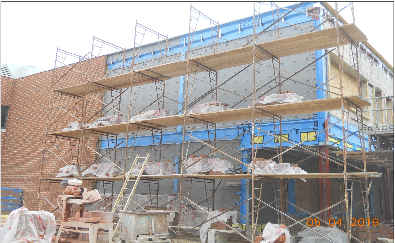
Pinelands Regional Sr. High School 6 Exterior Masonry Installation (Block A West)
