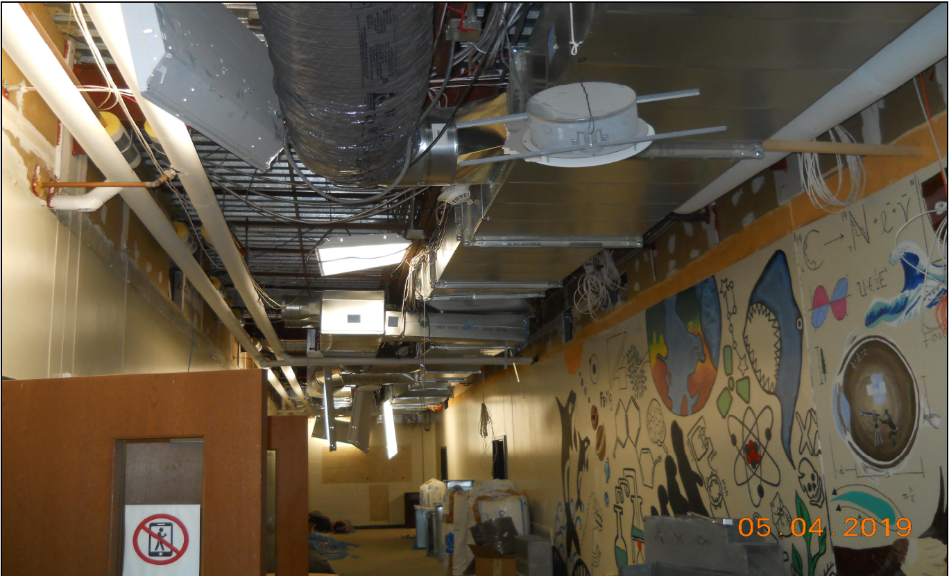
Pinelands Regional Sr. High School 6 HVAC Ductwork Installation (Block A South)
