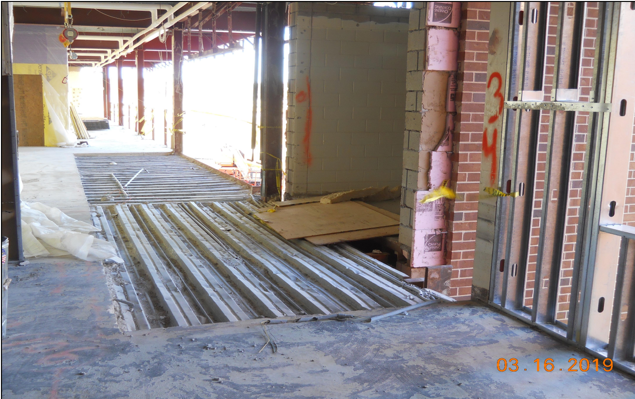
Pinelands Regional Sr. High School 6 2 nd Floor Concrete Floor Demo (Block A North)
