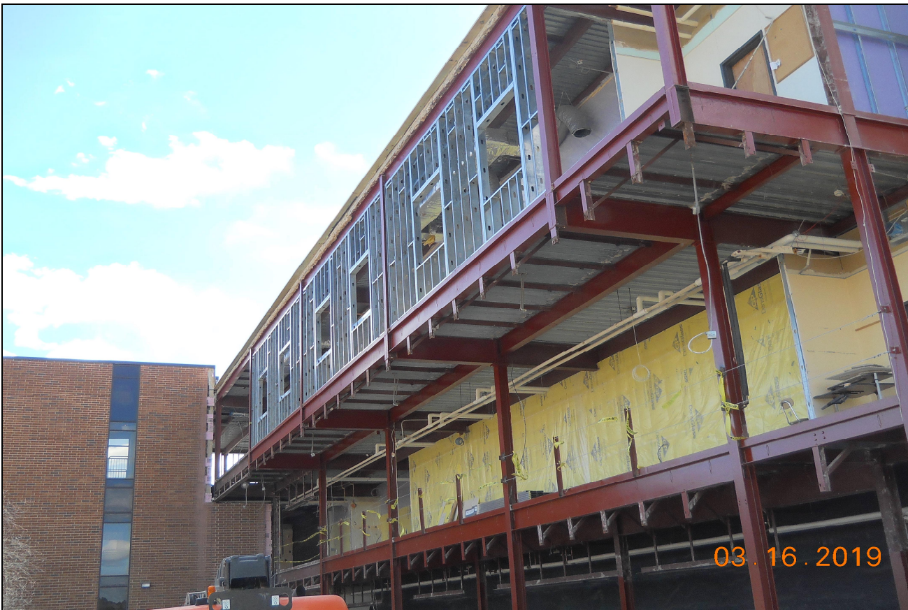
Pinelands Regional Sr. High School 6 Exterior Wall Structural Framing (Block A North)
