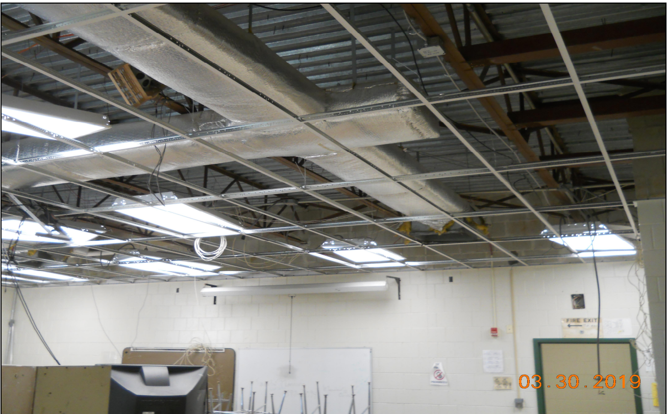
Pinelands Regional Sr. High School 6 Ceiling System Grid Installation (Block D Classroom)
