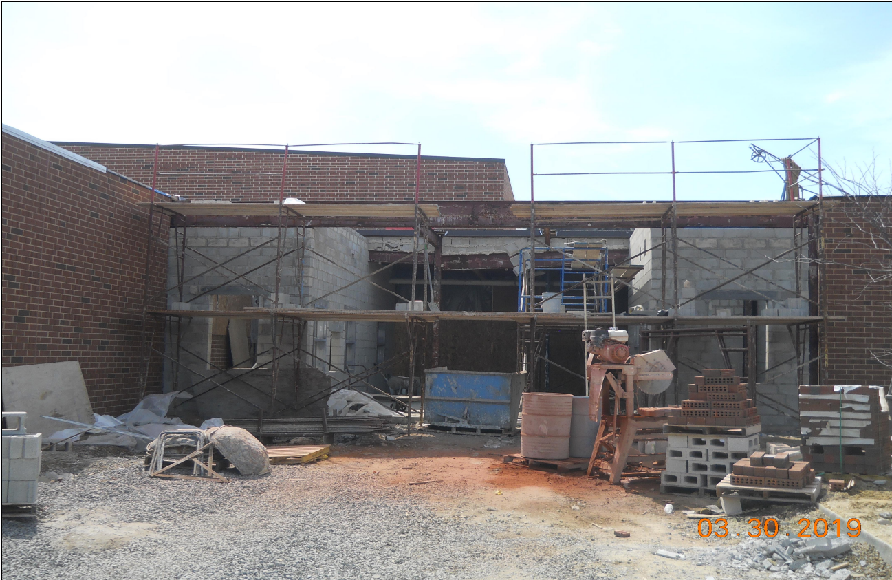
Pinelands Regional Sr. High School 6 Masonry Wall Installation (Main Entrance)
