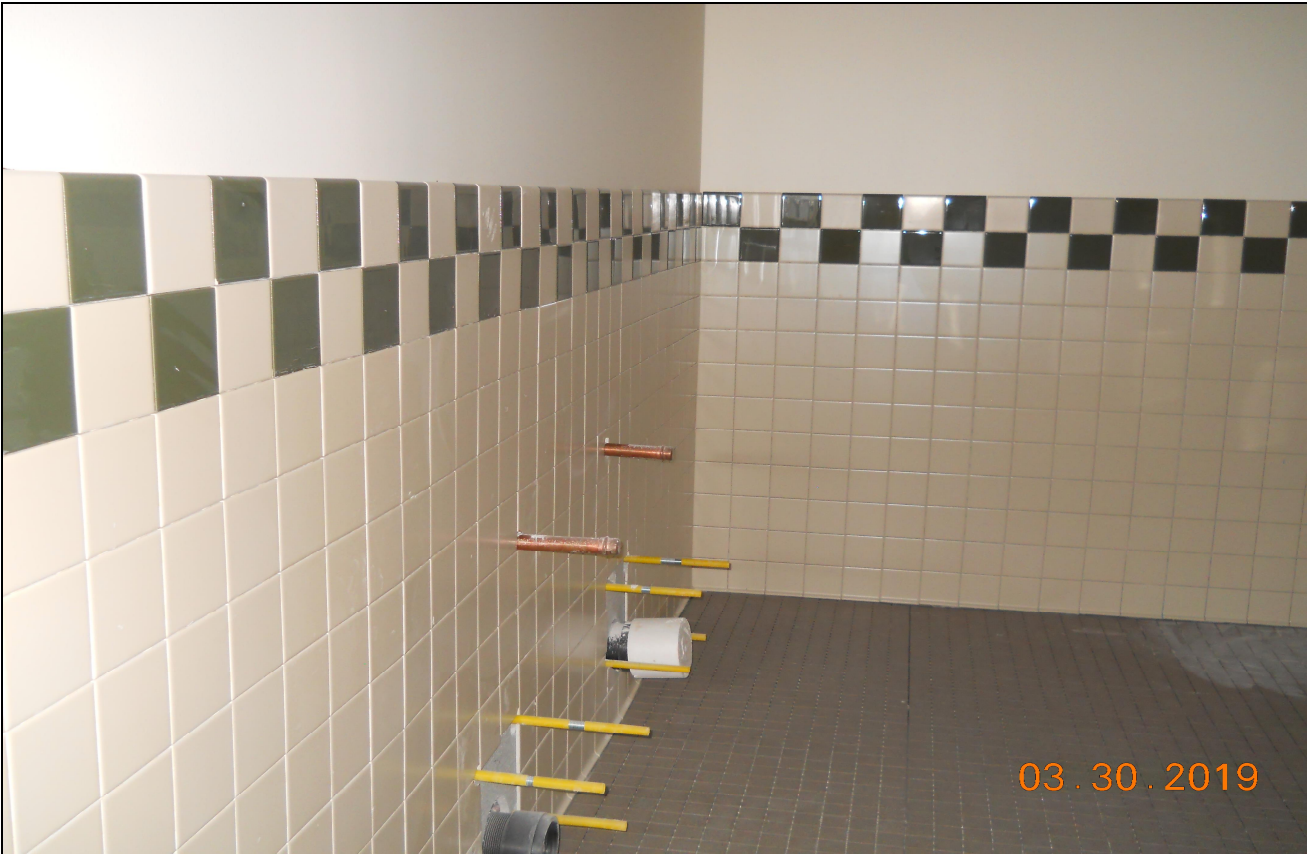
Pinelands Regional Sr. High School 6 Student Bathroom Ceramic Tile Installation (Block B)
