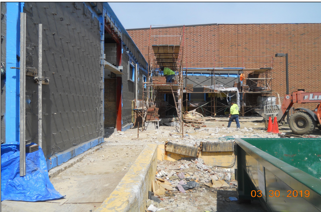
Pinelands Regional Sr. High School 6 Exterior Brick 6 Preparation & Installation (Block C East 6 Kitchen)
