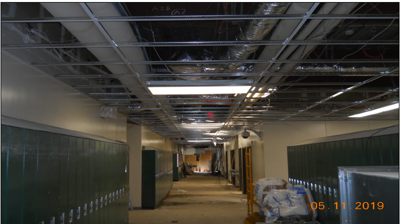
Pinelands Regional Sr. High School 6 Ceiling System & Lighting Installation (Block A North 6 Student Corridor 1 st Floor)
