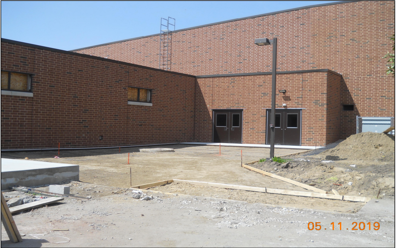
Pinelands Regional Sr. High School 6 Exterior Sidewalk Installation (Block C Rear)
