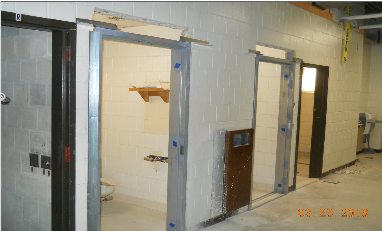
Pinelands Regional Sr. High School 6 Door Frame Installation (Block A South 6 Faculty Bathroom)
