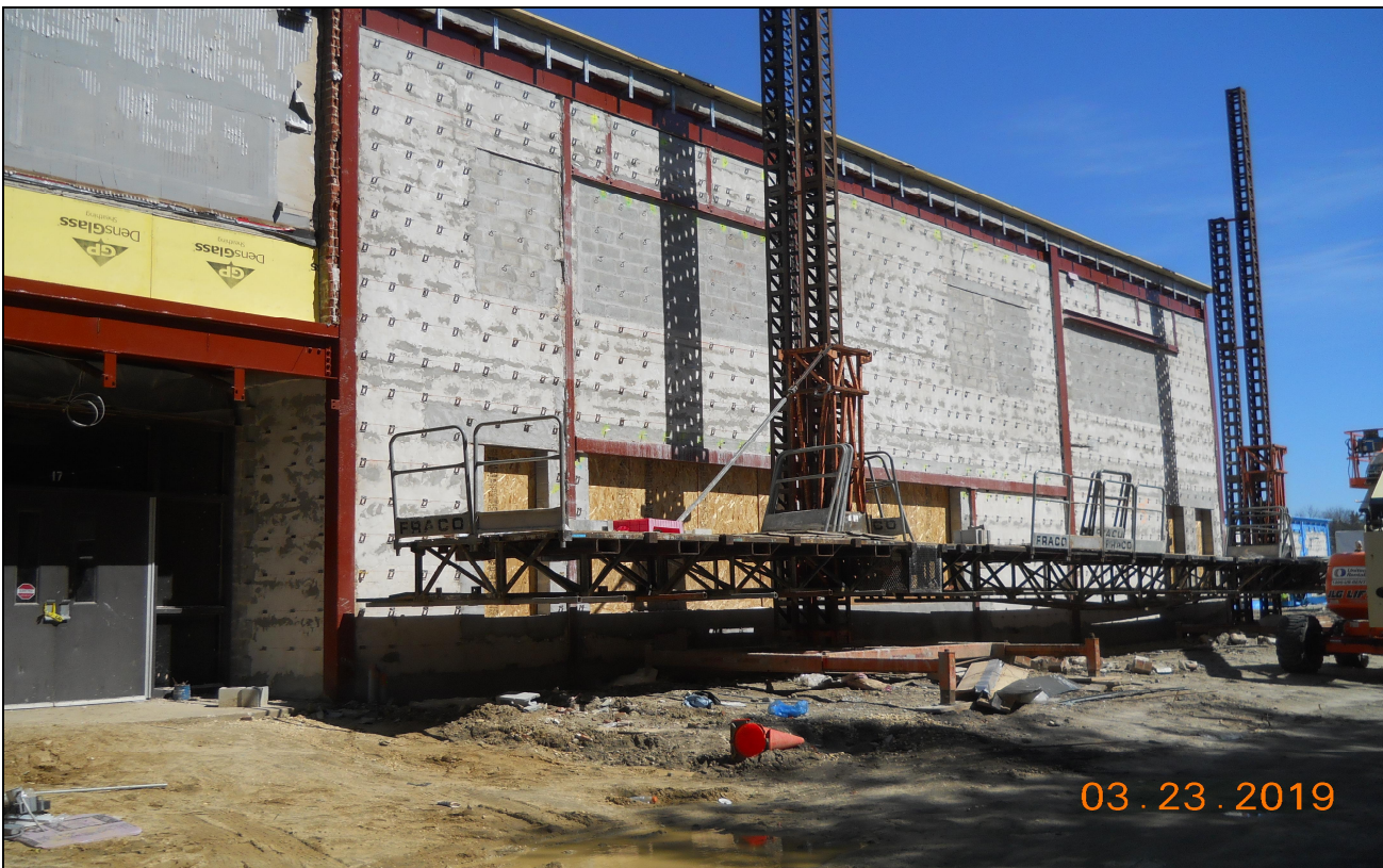
Pinelands Regional Sr. High School 6 Exterior Wall Preparation & Steel Installation (Block C South 6 Media Center)
