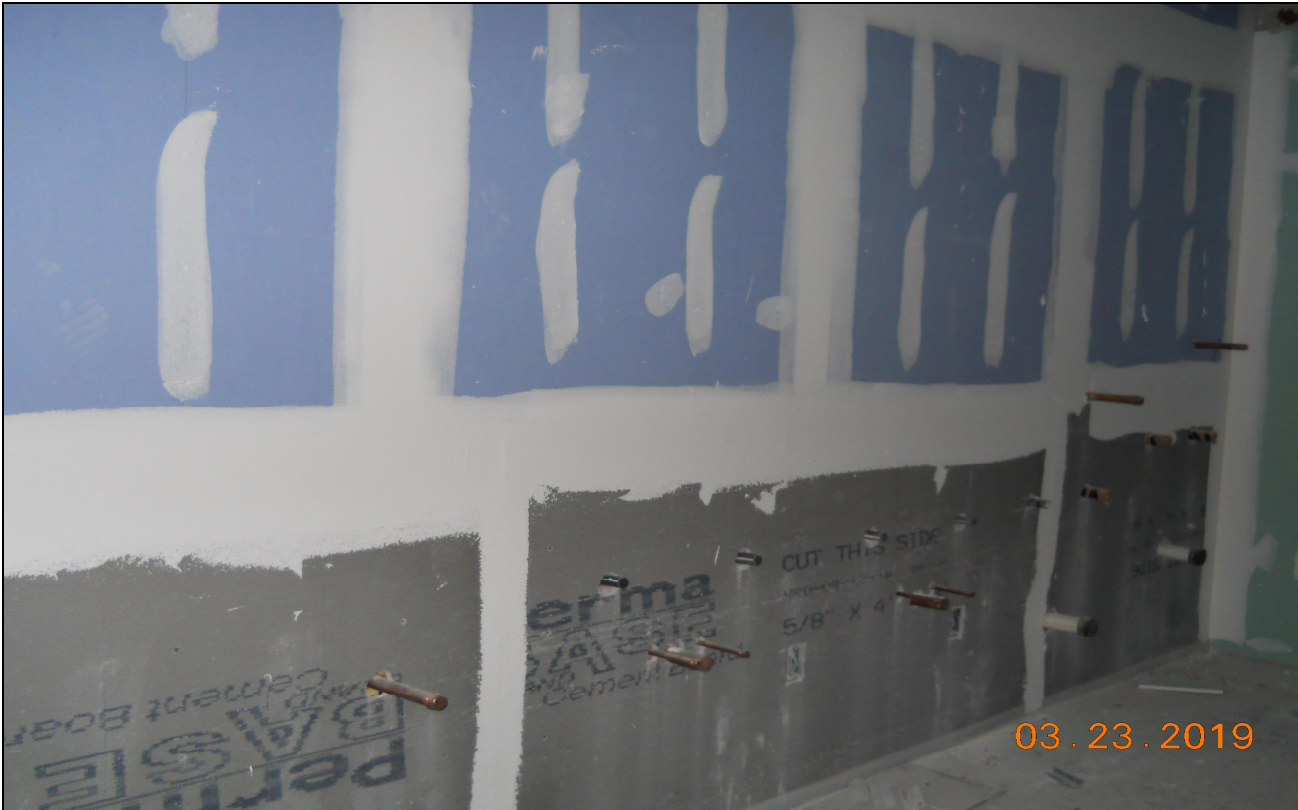
Pinelands Regional Sr. High School 6 Wall Preparation for Ceramic Tile (Block D Bathroom)
