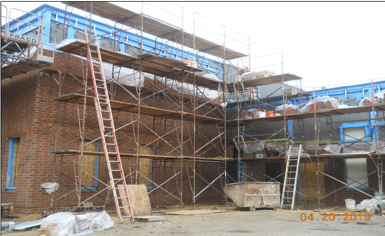
Pinelands Regional Sr. High School 6 Exterior Brick Installation (Block C South 6 Media Center & Cafe)
