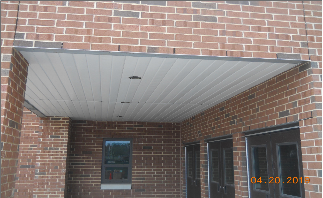
Pinelands Regional Sr. High School 6 Gym Entrance Canopy Soffit Installation (Block B)
