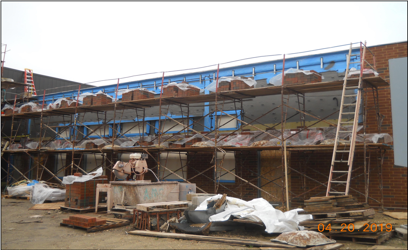
Pinelands Regional Sr. High School 6 Exterior Brick- Installation (Block C South 6 Cafeteria)
