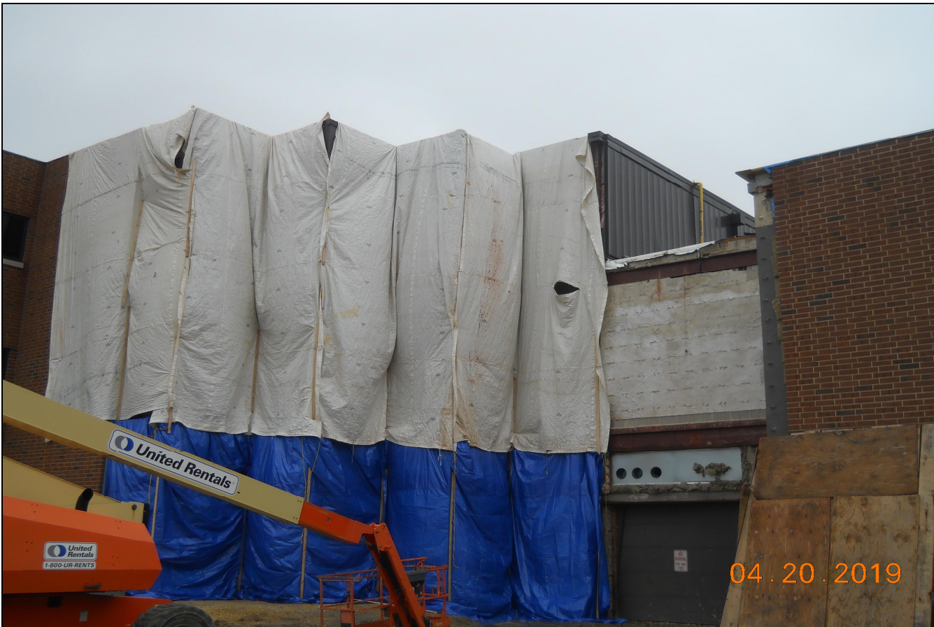
Pinelands Regional Sr. High School 6 Glazing Wall Protection (Block A West)
