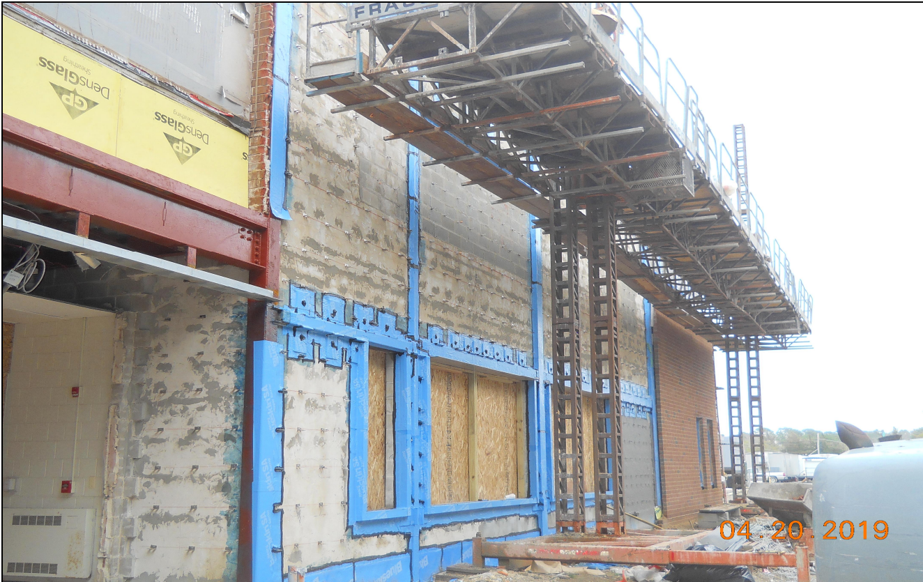
Pinelands Regional Sr. High School 6 Exterior Masonry Preparation & Installation - (Block A South Media Center)
