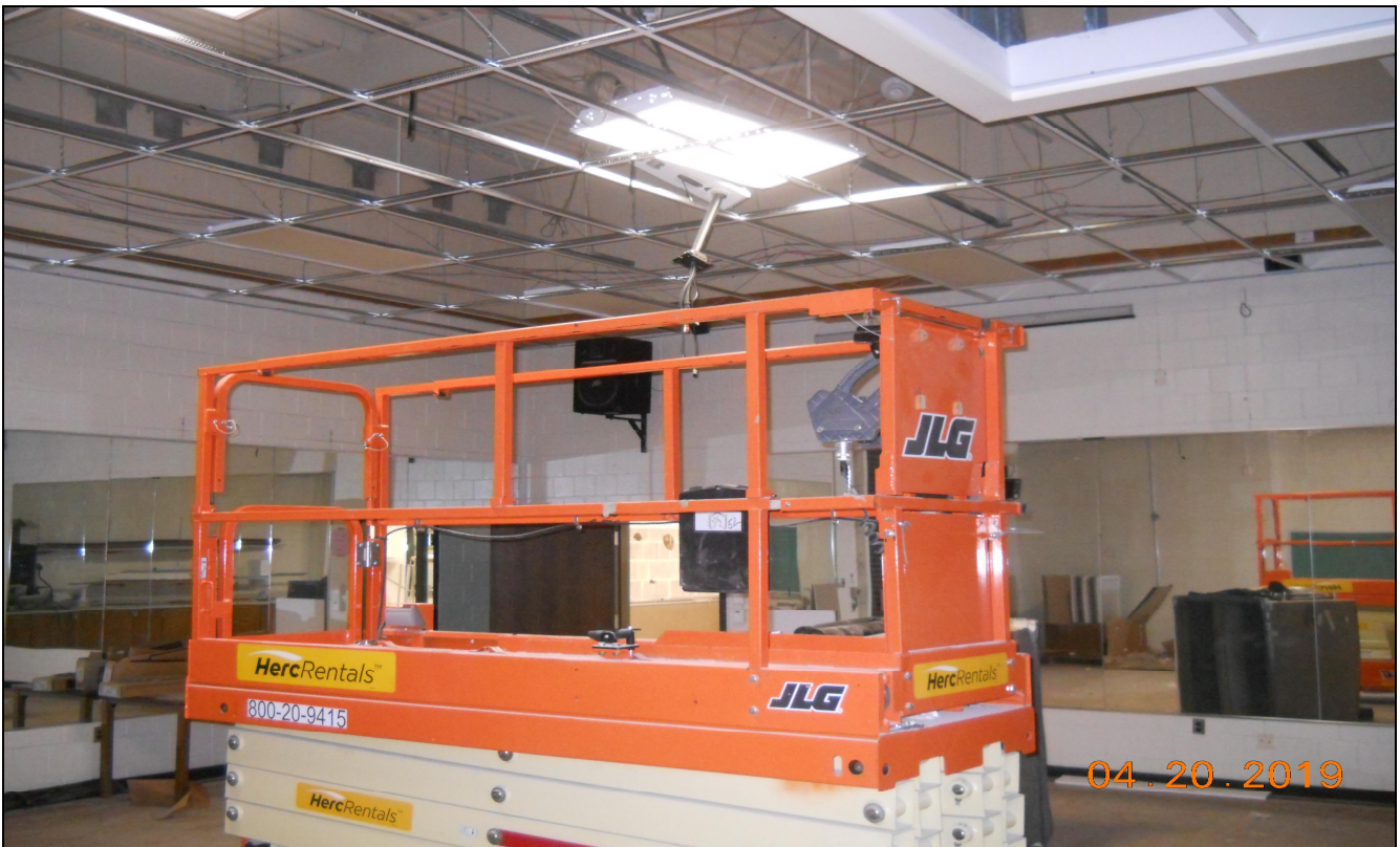
Pinelands Regional Sr. High School 6 Drama Classroom Ceiling grid installation (Block D)
