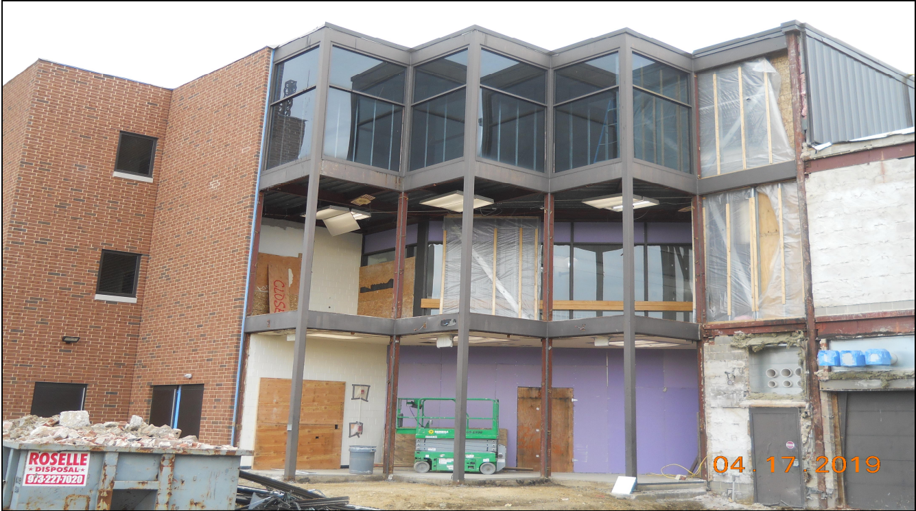
Pinelands Regional Sr. High School 6 Exterior Glazed Curtain Wall Demolition (Block A West)
