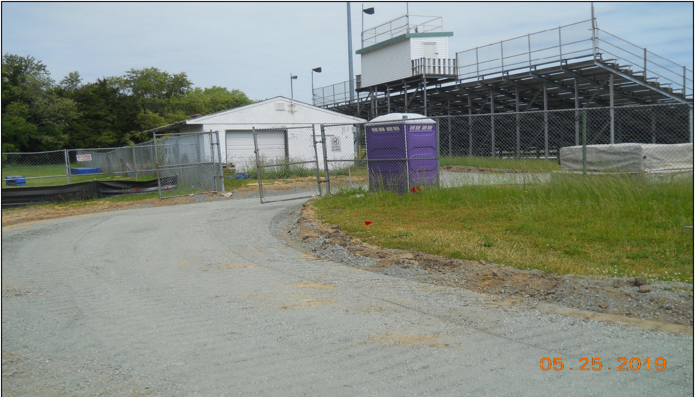
Pinelands Regional Sr. High School 6 Pavement Preparation (Walkway Sub-base)
