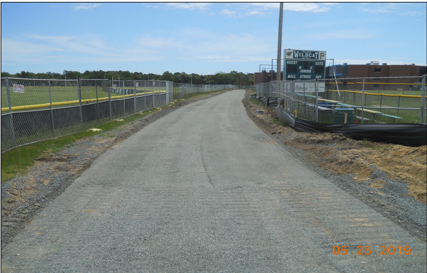
Pinelands Regional Sr. High School 6 Pavement Preparation (Walkway Sub-base)
