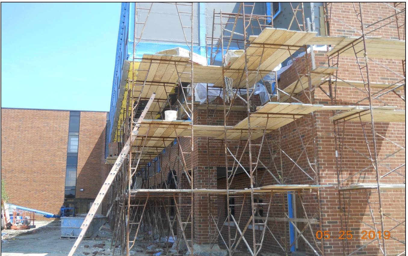
Pinelands Regional Sr. High School 6 Exterior Masonry Installation (Block A North)
