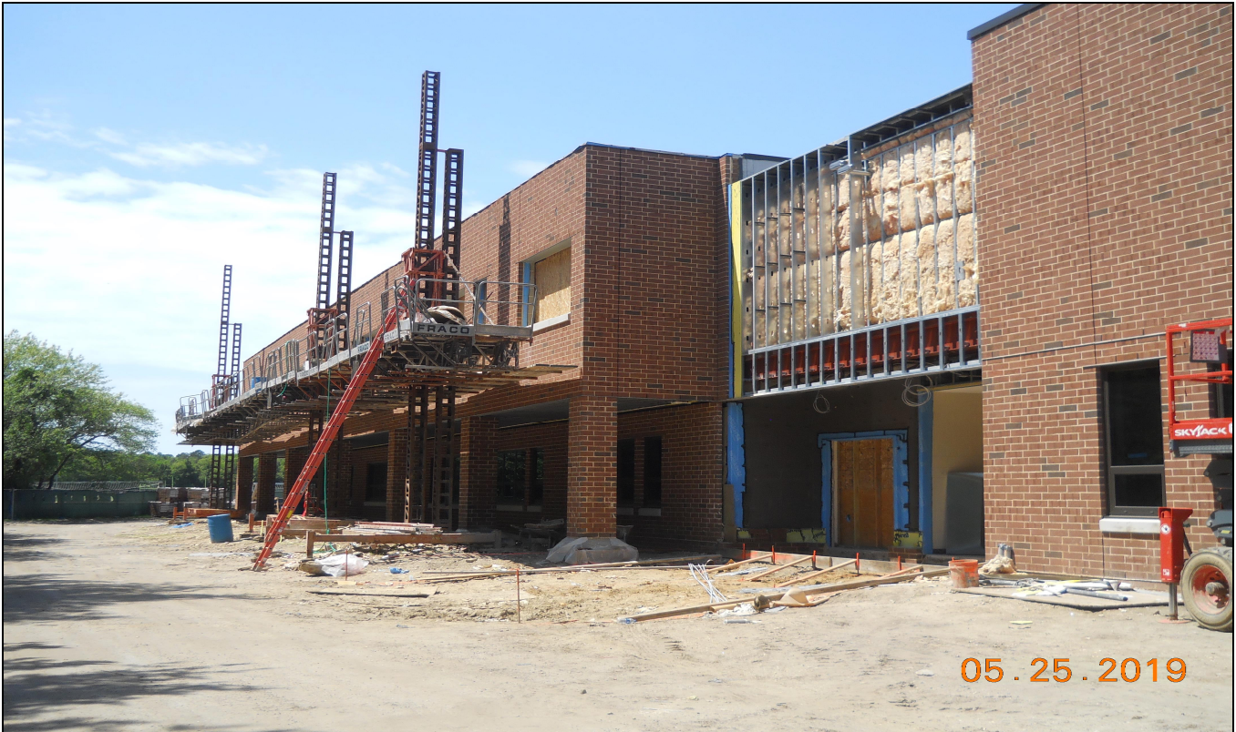
Pinelands Regional Sr. High School 6 Exterior Brick & Window Installation (Block A - South)
