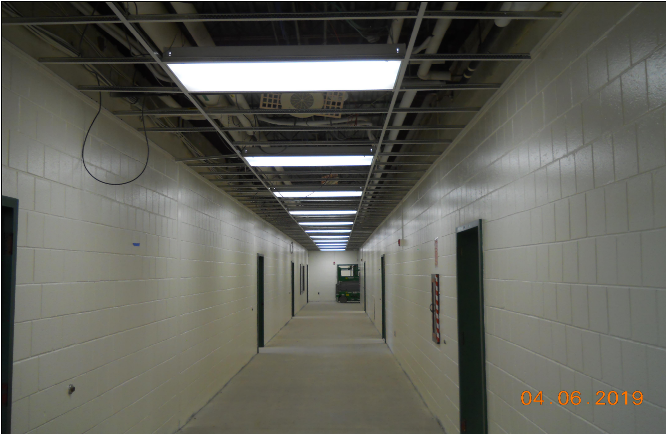
Pinelands Regional Sr. High School 6 Student Corridor 6 Ceiling Grid & Lighting 6 Installation (Block D)
