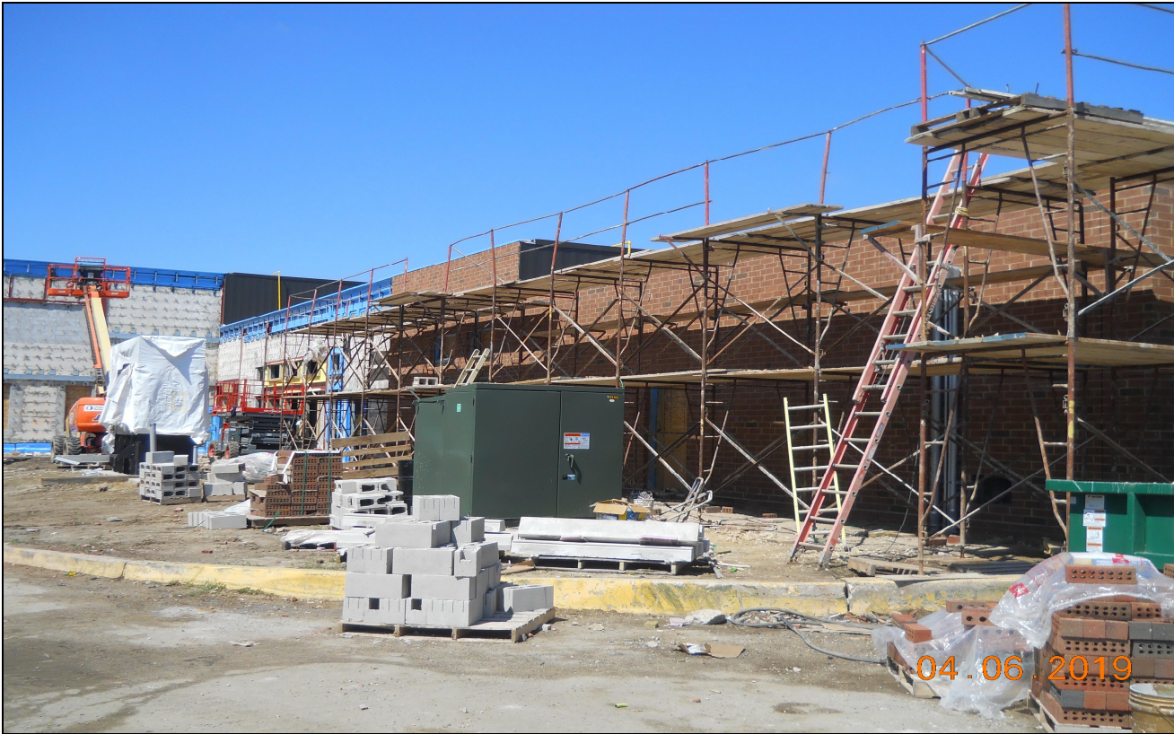
Pinelands Regional Sr. High School 6 Exterior Brick- Installation (Block C South 6 Cafeteria)
