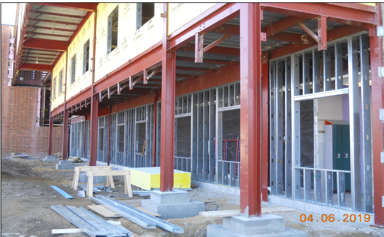
Pinelands Regional Sr. High School 6 Exterior Wall Structural Framing (Block A North)
