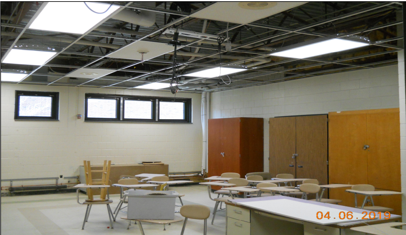
Pinelands Regional Sr. High School 6 Classroom 6 Ceiling Grid & Lighting 6 Installation (Block D)
