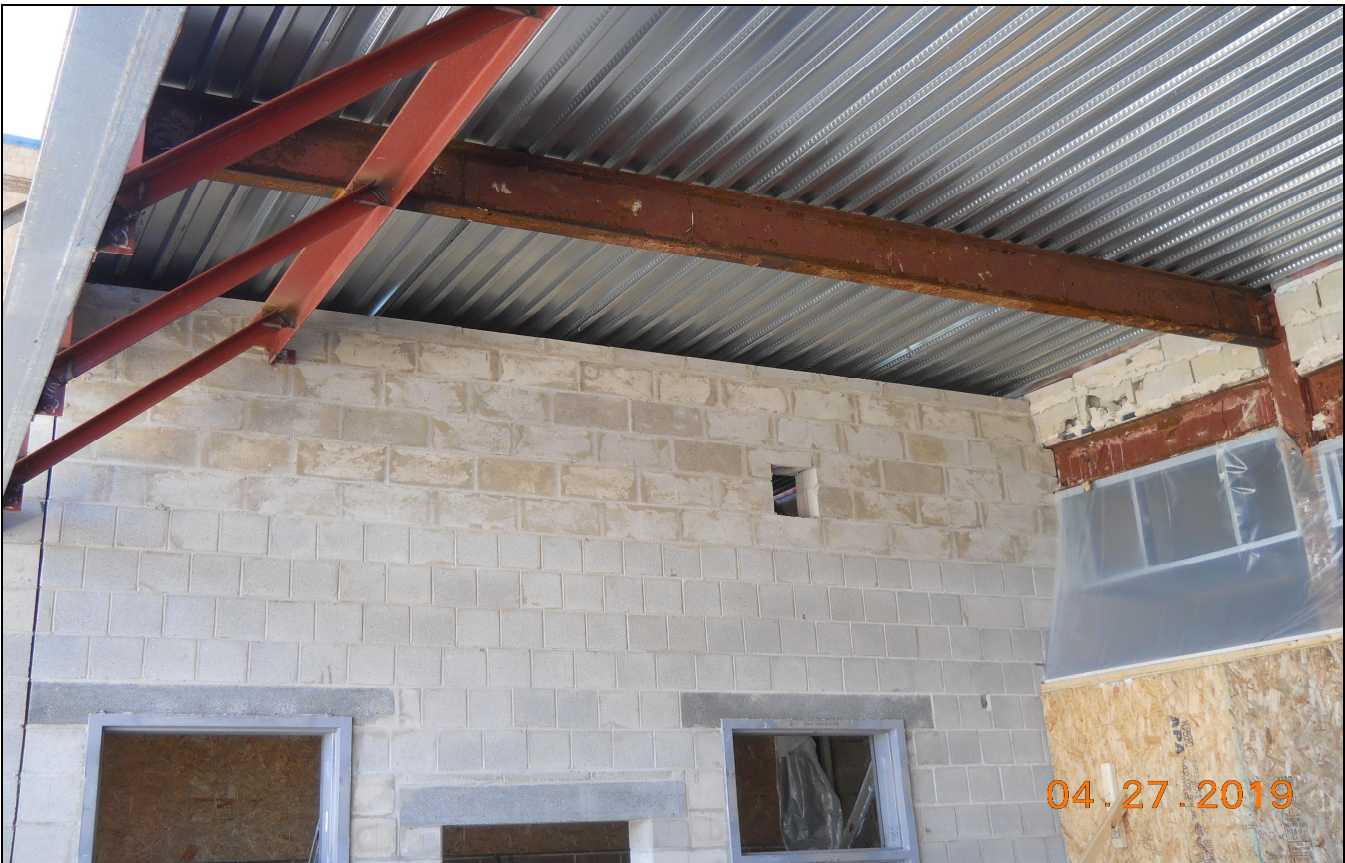
Pinelands Regional Sr. High School 6 Structural Steel Roof Decking (Block B Main Entrance)
