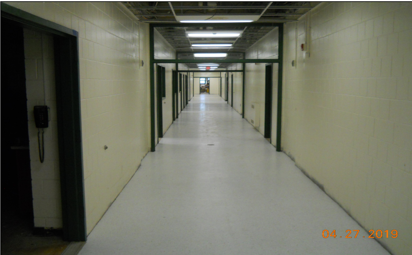
Pinelands Regional Sr. High School 6 VCT Flooring Installation (Block D Corridor)
