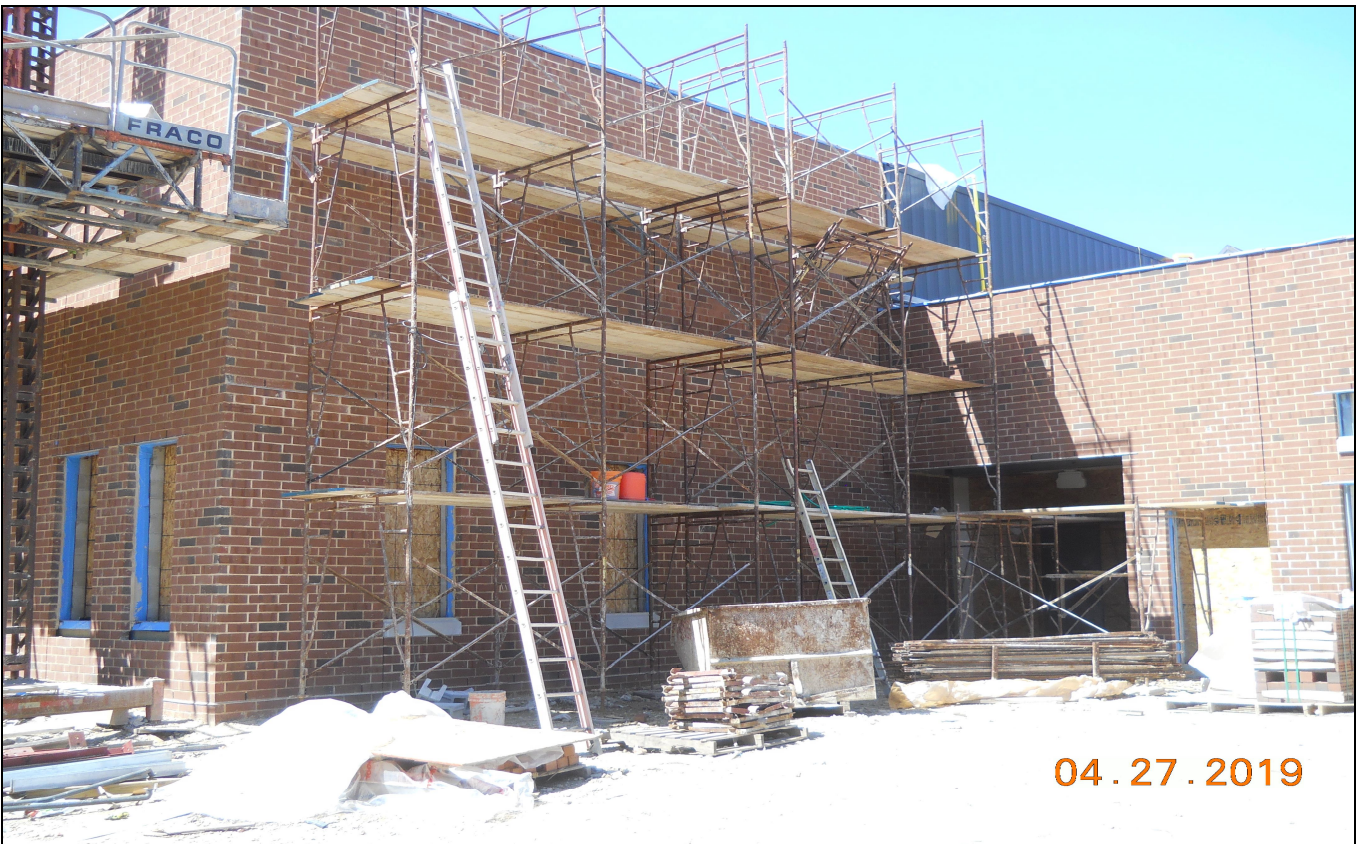
Pinelands Regional Sr. High School 6 Exterior Brick Installation (Block C South 6 Media Center & Cafe)
