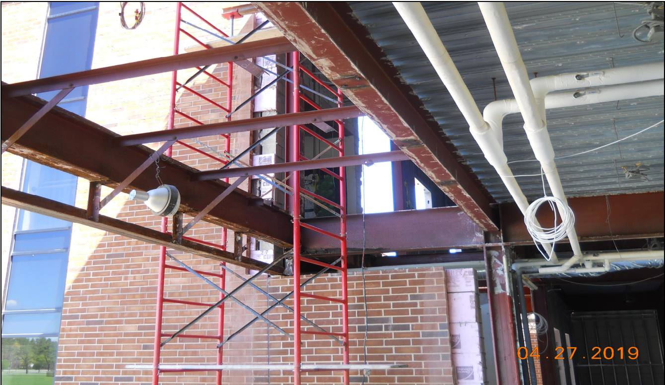
Pinelands Regional Sr. High School 6 Structural Steel Restoration (Block A North)
